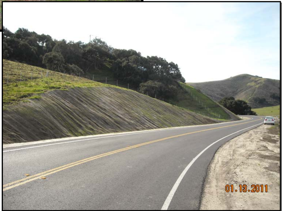
Harris Grade Road – Completed Project (Looking South)
