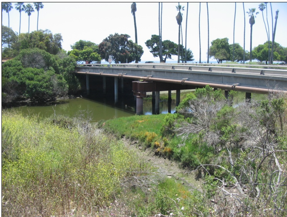
Photo 2.3. East side view of bridge.
