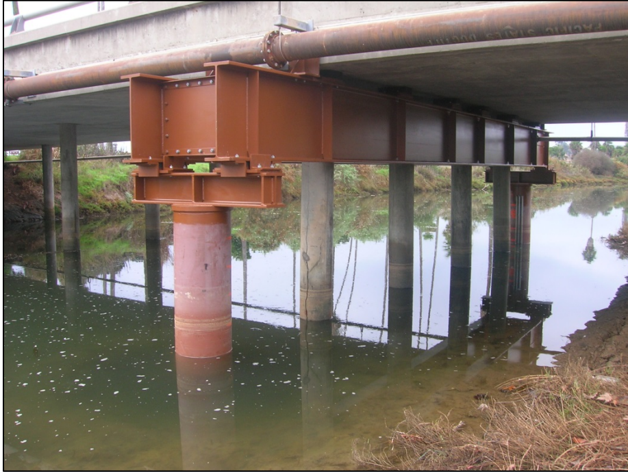
Photo 2.6. Completed temporary pier support.
