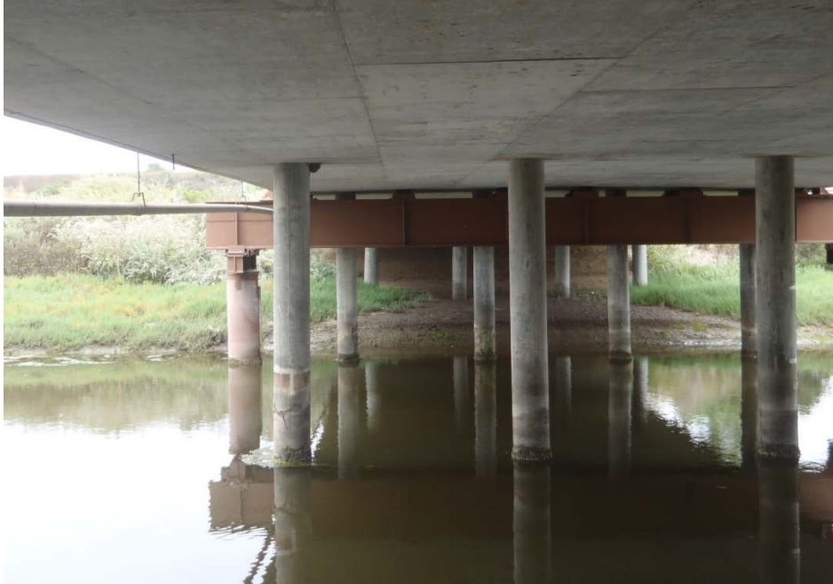
Photo 2.4. View of existing pilings.
