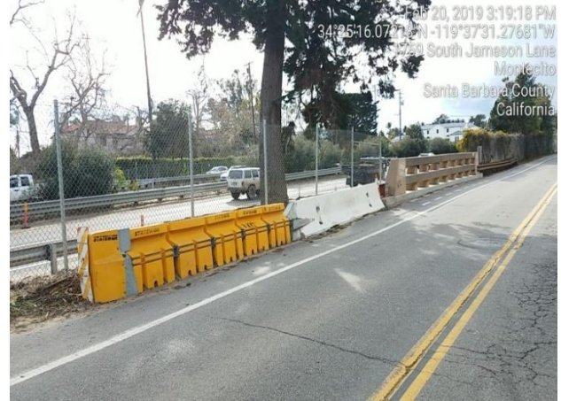
Left photo: Oak Creek BR 51C-0343 damaged bridge approach railing during emergency opening operations. Right photo: Existing Conditions - Temporary crash cushion and barricade at Oak Creek BR 51C-0343.
