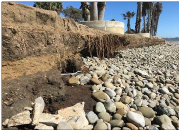
Figure 2. The 2015-2016 El Nino overwhelmed cobble berm protection at Surfers' Point, exposing park facilities to damage (left); in response, the City expended $430,000 to install a 260-foot long 13.5 feet tall emergency rock revetment and cobble replenishment. The project is not yet completed.
