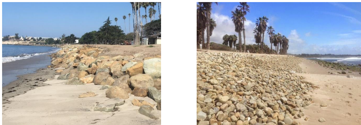
Figure 1. Goleta Beach revetment (left) and Surfers' Point C-Street expansion cobble berm (right) Surfers' Point Photo source: https://toolkit.climate.gov/case-studies/restoring-surfers-point-partnerships-persistence-pays
