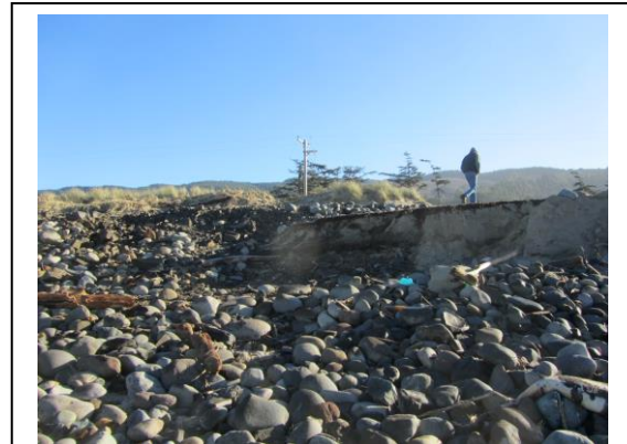
Cape Lookout State Park in Oregon suffered erosion damage in fall and winter of 2016 along the cobble and dune beach, destroying a segment of park access road. Note cobbles and eroded dunes in background. Oregon Shores Conservation Coalition, October 2016
