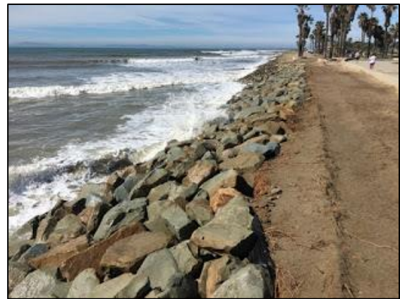
Figure 2. The 2015-2016 El Nino overwhelmed cobble berm protection at Surfers' Point, exposing park facilities to damage (left); in response, the City expended $430,000 to install a 260-foot long 13.5 feet tall emergency rock revetment and cobble replenishment. The project is not yet completed.
