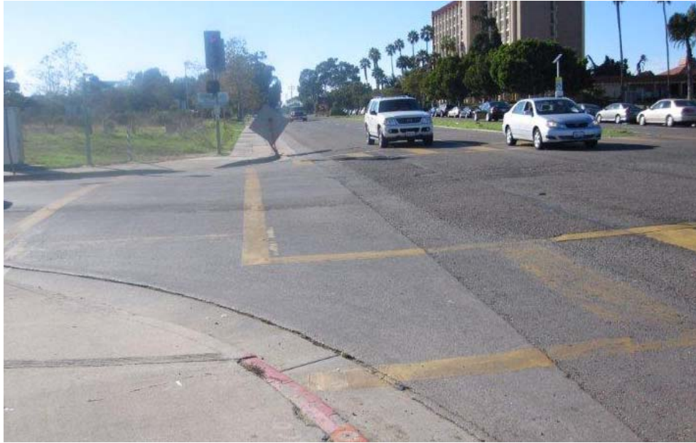
Typical road to be rehabilitated
