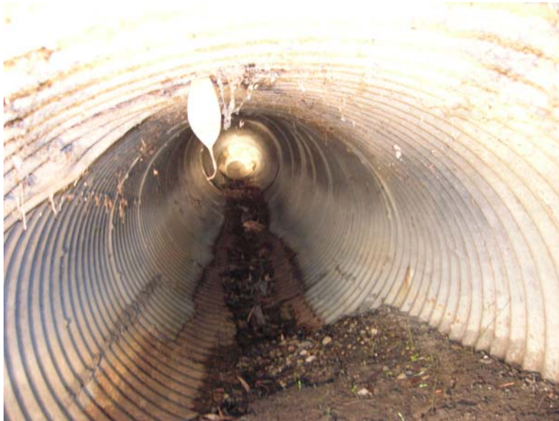
Existing Pipe Culvert under Alston Road
