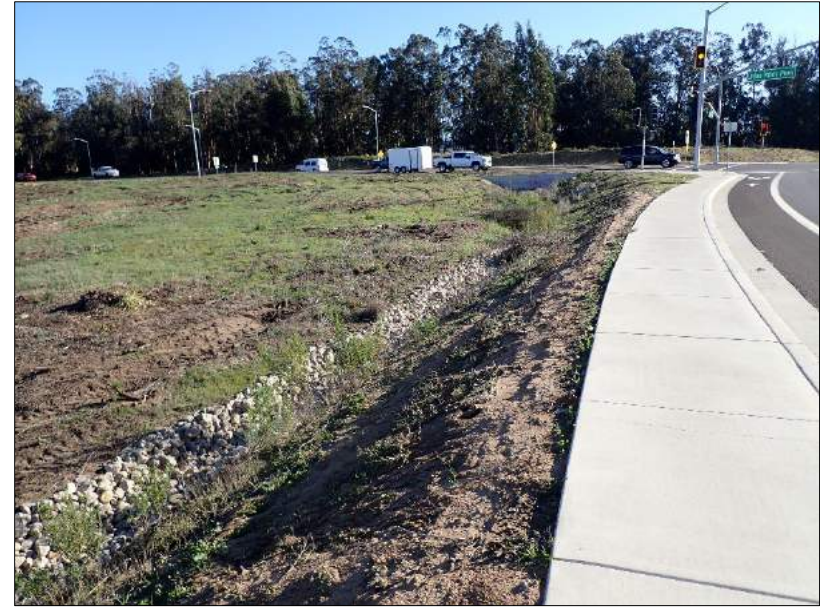
Photo 22: View south at constructed rocky ditch roadside drainage management system on Orcutt Road at UVP. 12/17/2021
