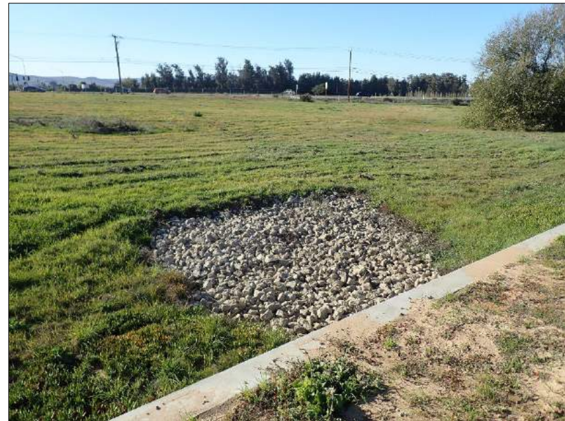
Photo 24: View west at drainage rock at culvert under Orcutt Road. No continued drainage pattern. 12/17/2021
