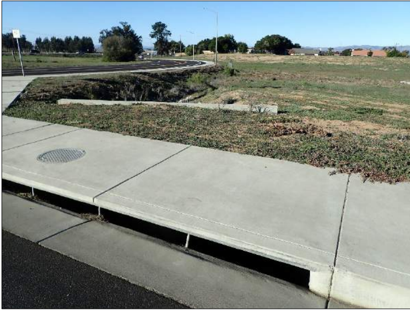
Photo 21: View north at stormdrain inlet and constructed ditch drainage management system on UVP at Orcutt Road. 12/17/2021
