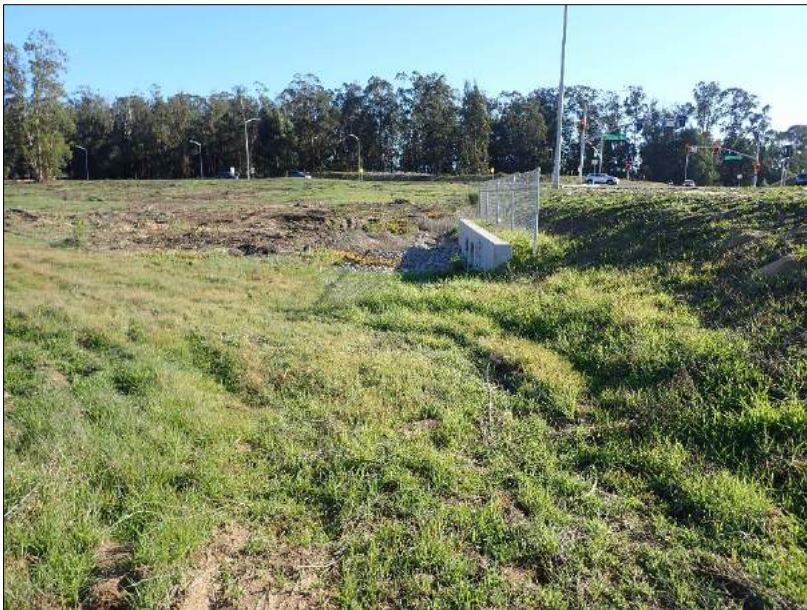
Photo 23: View south at constructed ditch drainage management system and culvert under Orcutt Road. 12/17/2021
