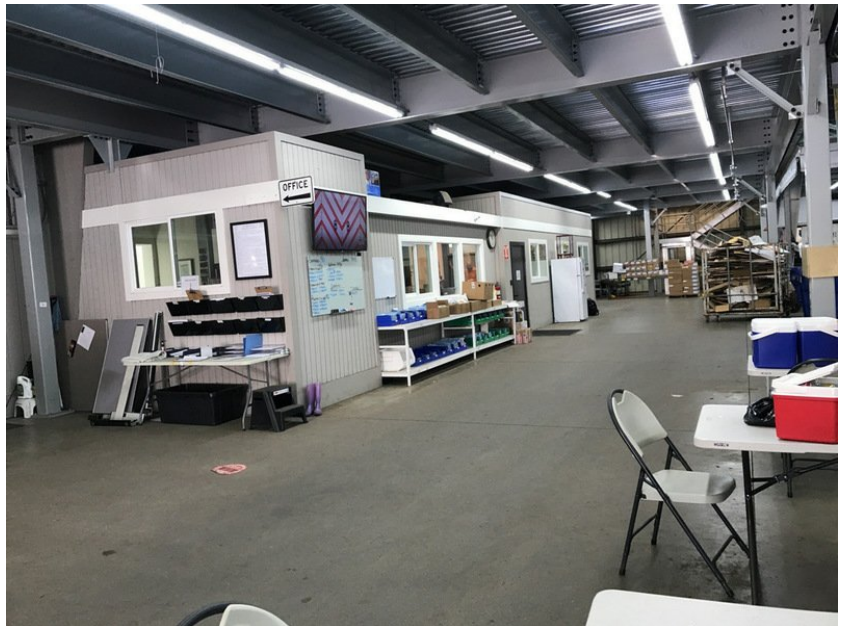
As built offices.
