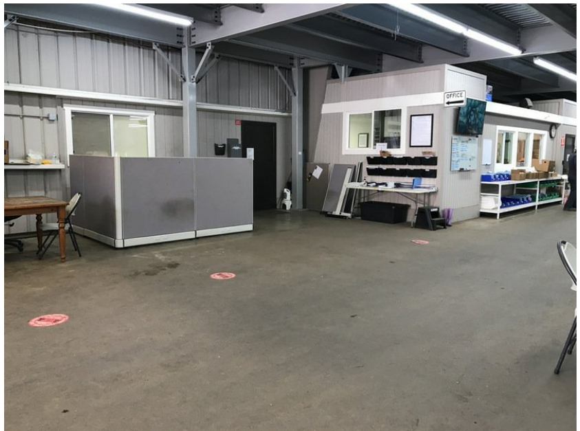
As built offices.
