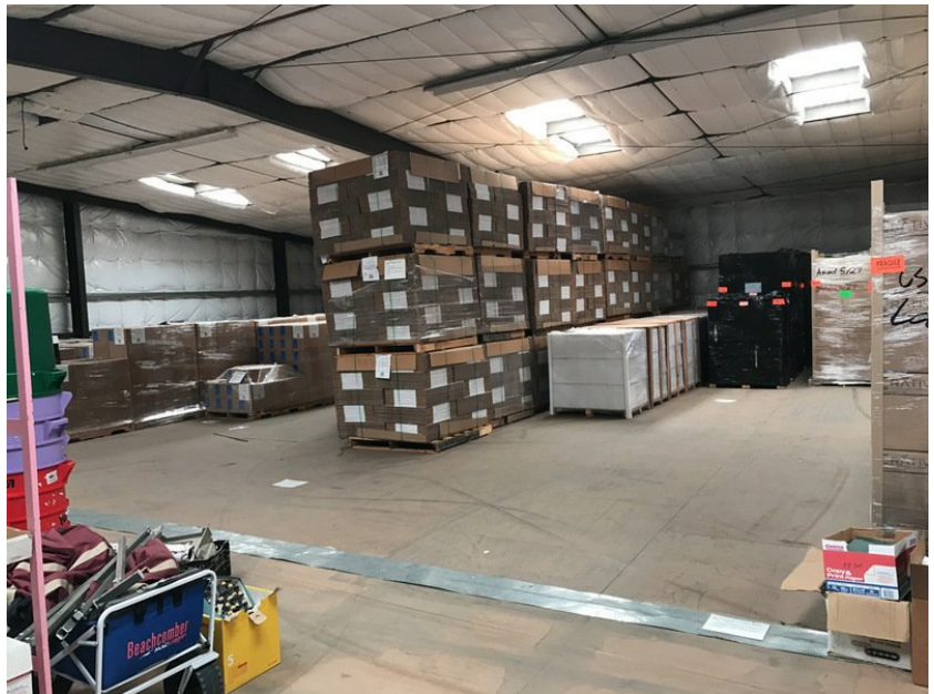
Storage in un-permitted second story to be removed. Completed 9/13/2021
