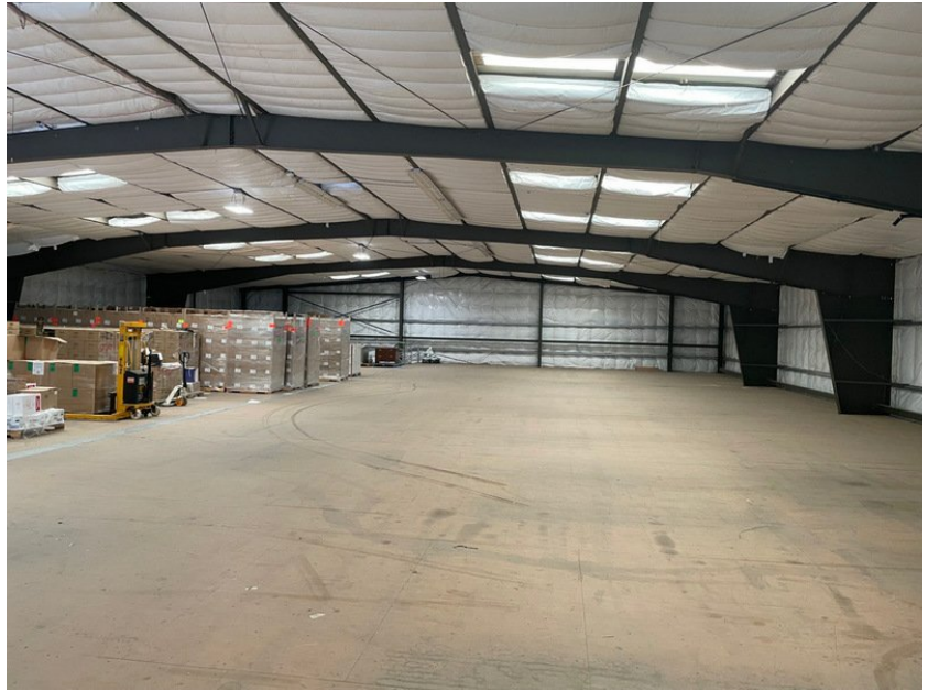
Cleared second floor storage
