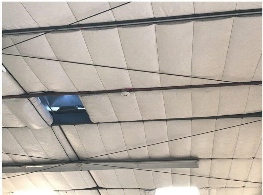
Permit for Fire alarm system and additional work required.
