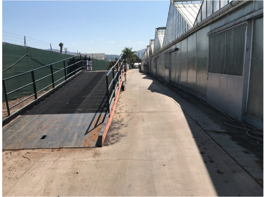
Access road on the north side of the building
