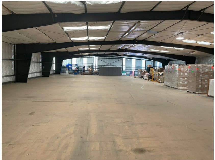
Cleared 2nd floor storage
