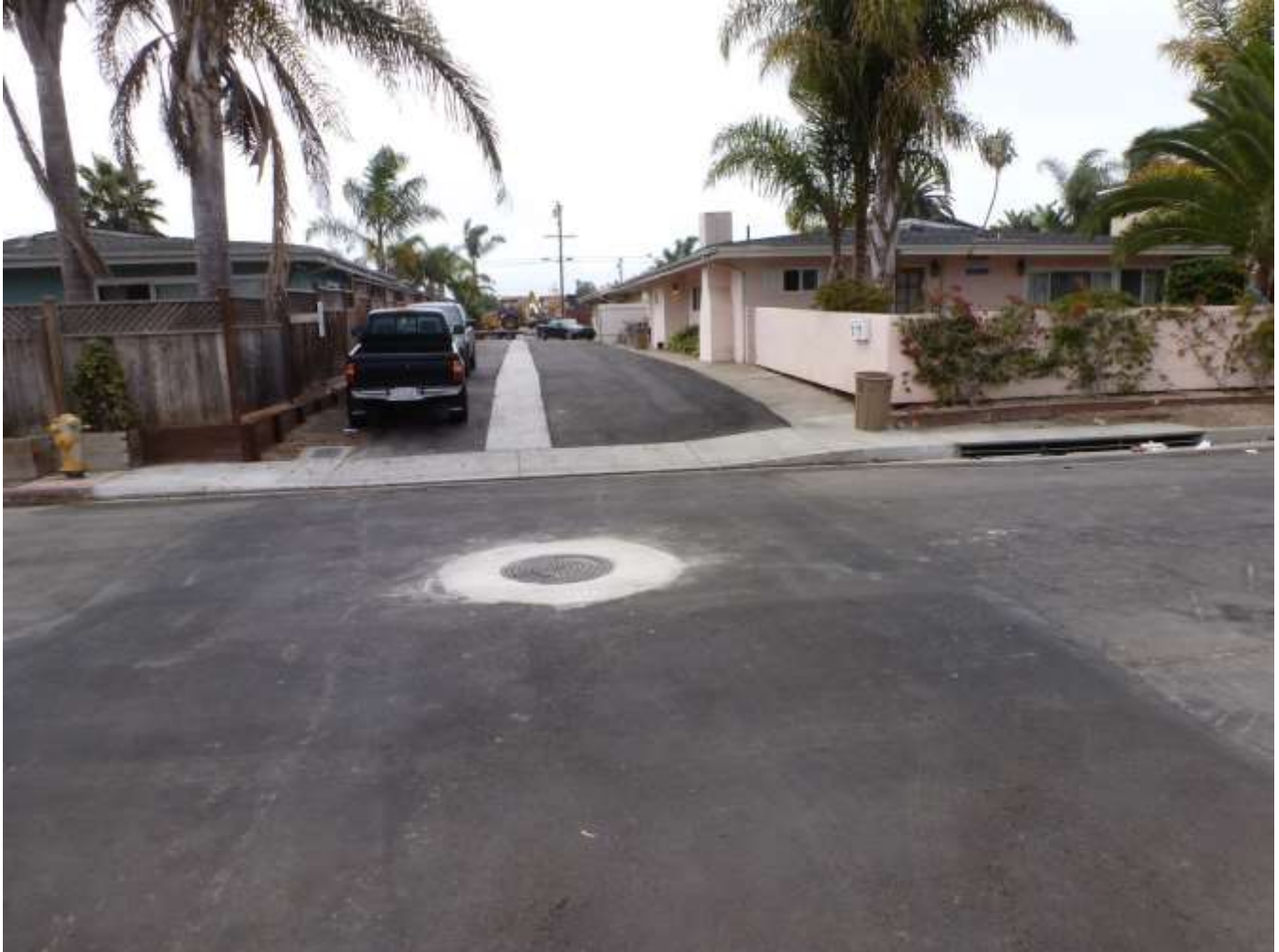
Isla Vista Storm Drain Improvement Project – Trigo Road looking South
