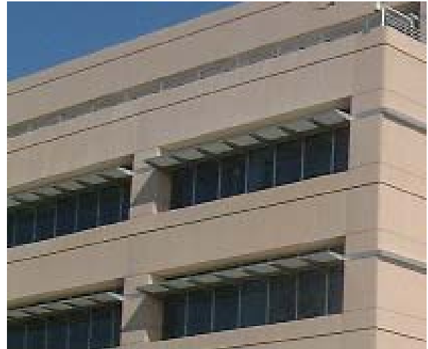
Figure 2-11. Exterior Light Shelves at the U.S. EPA Regional Headquarters, Kansas City, Kansas. The exterior light shelves reflect natural light upward across the interior ceilings, thereby projecting light deeper into the building. The light shelves also help to reduce glare and increase the visual comfort of the interior spaces for the building occupants. (Photo: Don Horn)
