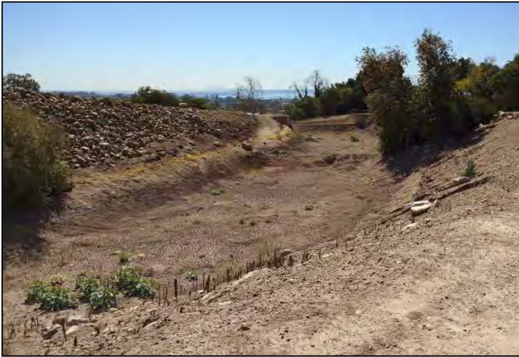
PHOTOGRAPH 5.9-1 Santa Monica Creek Debris Basin Plunge Pool Below Basin
