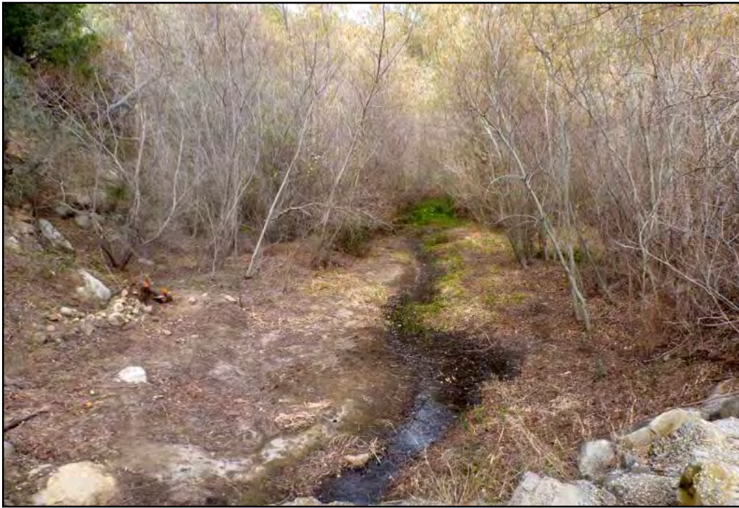
PHOTOGRAPH 5.4-3 San Ysidro Creek Debris Basin Looking Upstream
