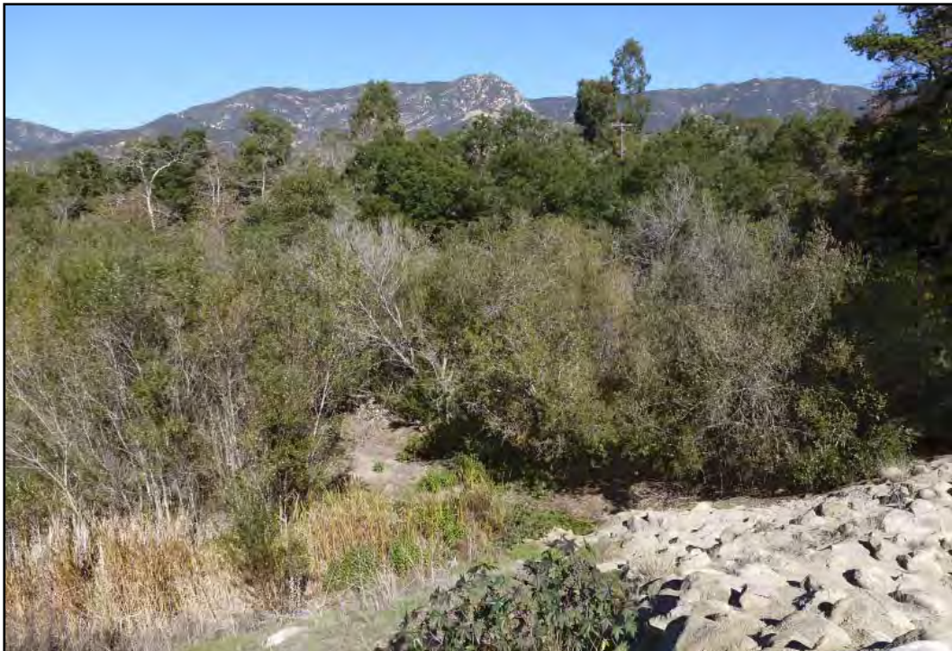
PHOTOGRAPH 5.11-2 Lower West Toro Canyon Creek Debris Basin
