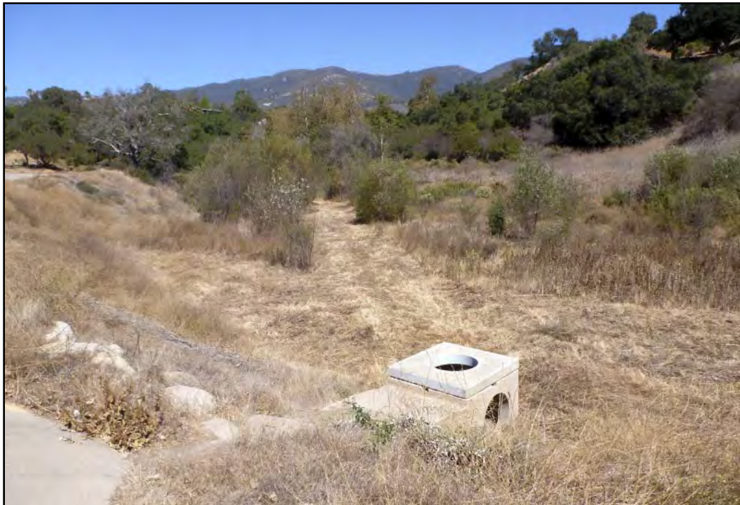
PHOTOGRAPH 5.7-2 San Antonio Creek Debris Basin
