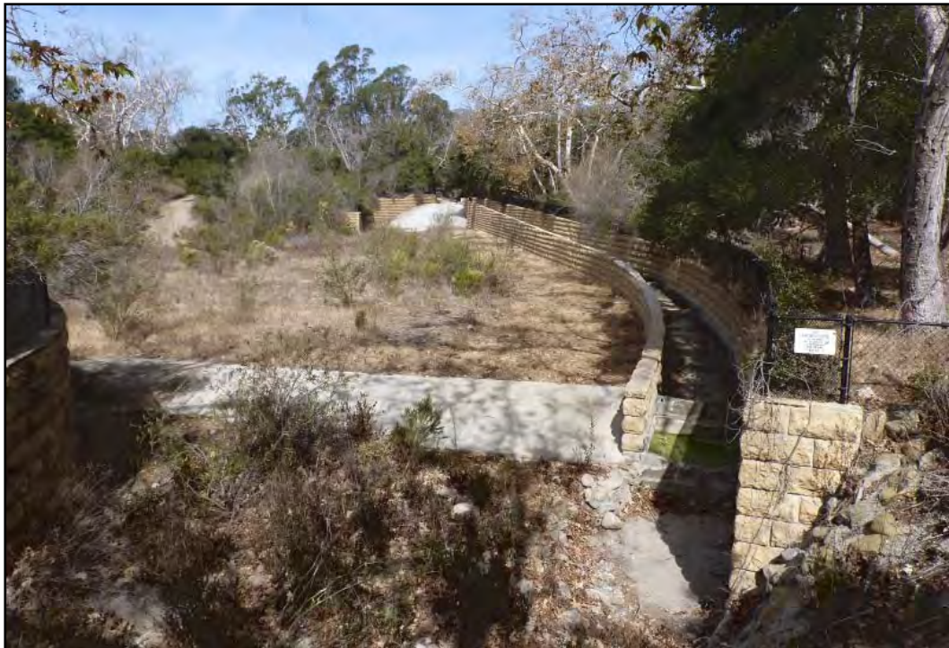
PHOTOGRAPH 5.5-2 Montecito Creek Debris Basin
