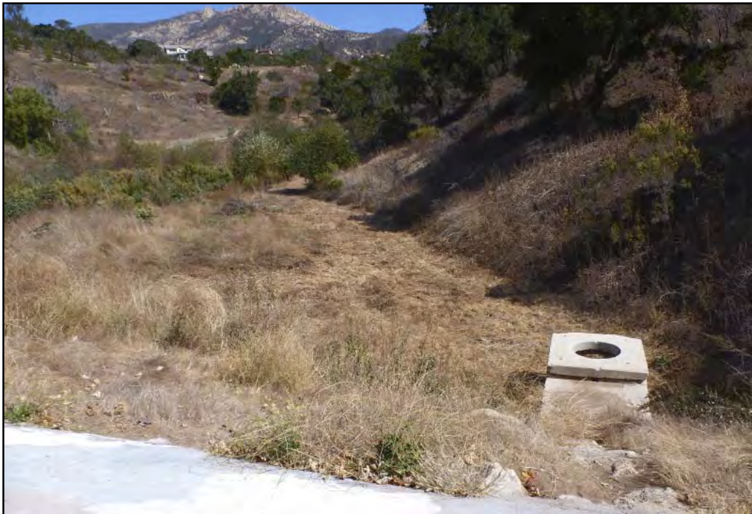
PHOTOGRAPH 5.8-2 San Roque Creek Debris Basin
