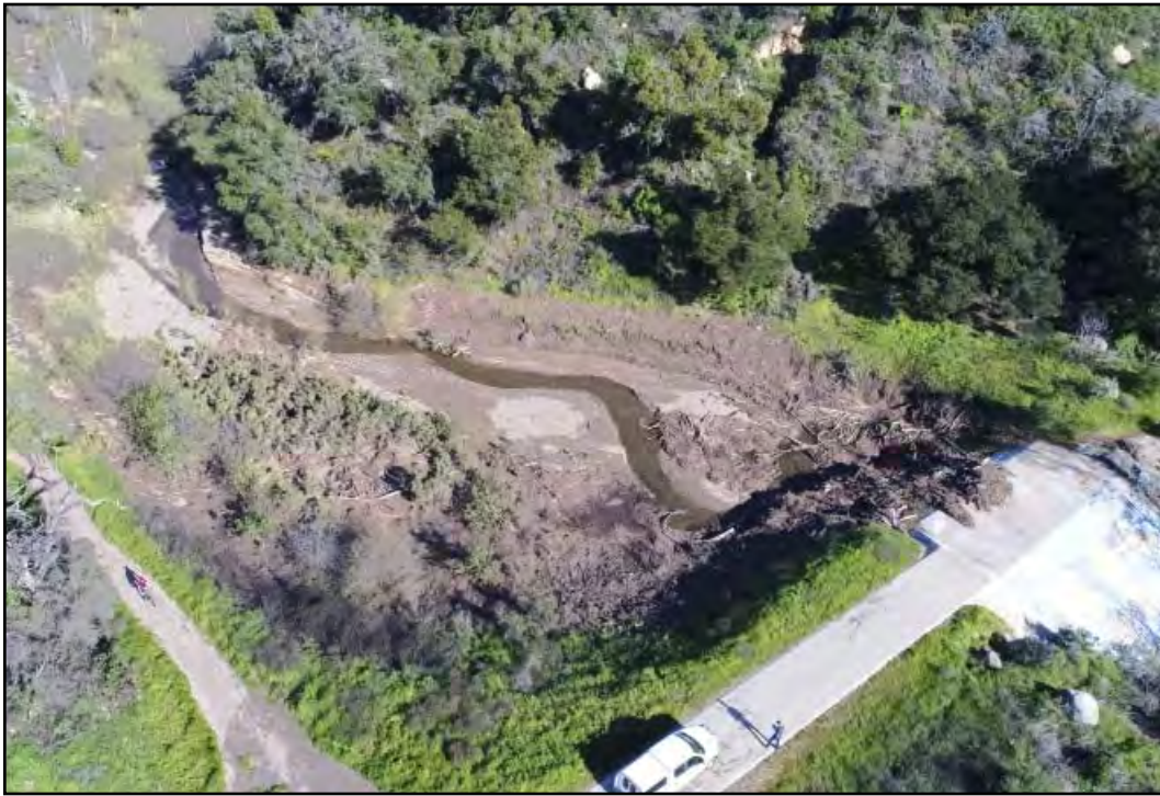
PHOTOGRAPH 5.8-1 San Roque Creek Debris Basin
