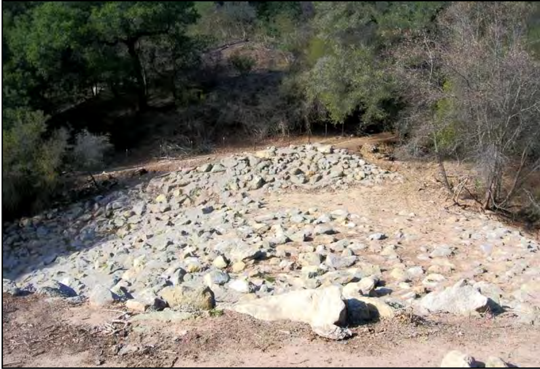
PHOTOGRAPH 4.3-3 Maria Ygnacio Creek, Main Branch Debris Basin Embankment
