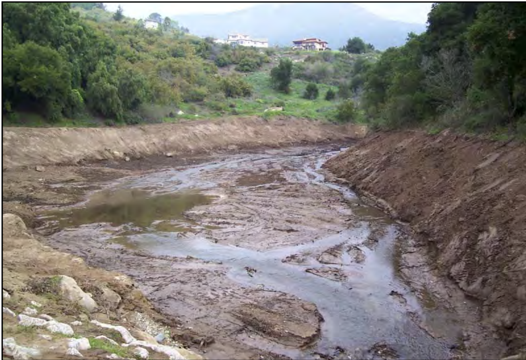
PHOTOGRAPH 2-1 San Roque Creek 2005 Desilting
