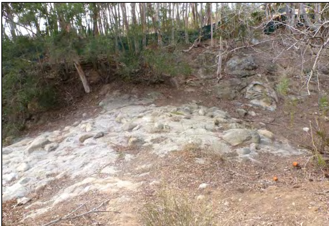
PHOTOGRAPH 5.4-2 San Ysidro Creek Debris Basin Embankment
