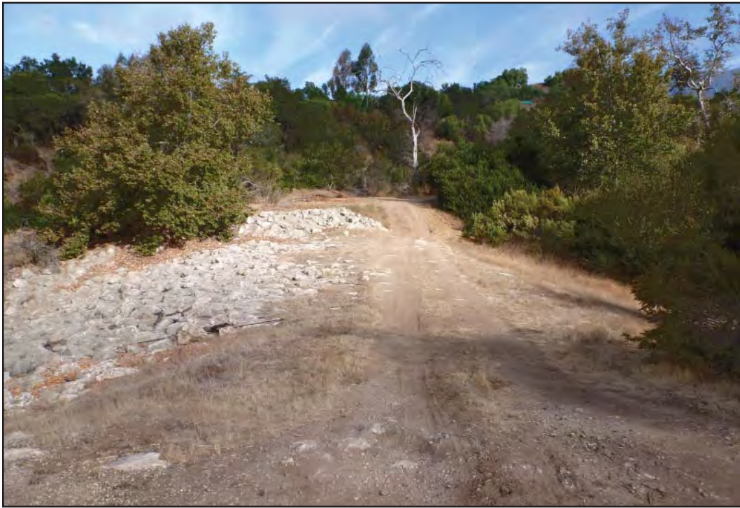
PHOTOGRAPH 4.2-1 Maria Ygnacio Creek, East Branch Debris Basin Embankment
