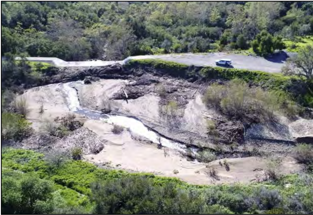
PHOTOGRAPH 5.7-1 San Antonio Creek Debris Basin
