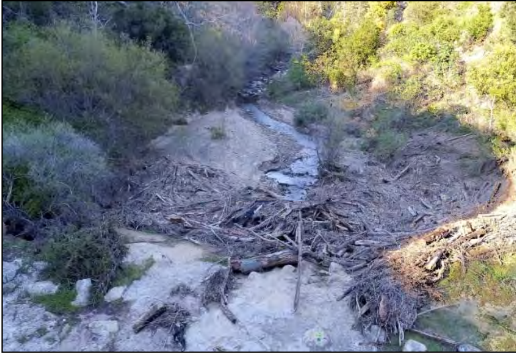
PHOTOGRAPH 5.4-1 Mission Creek Debris Basin
