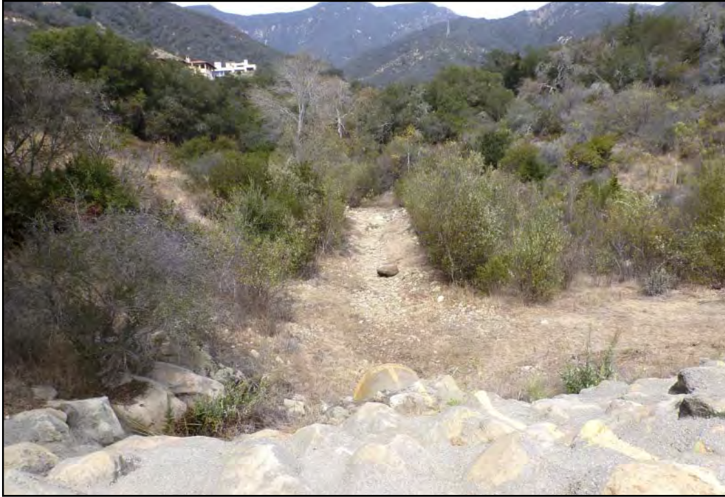
PHOTOGRAPH 5.10-1 East Toro Canyon Creek Debris Basin
