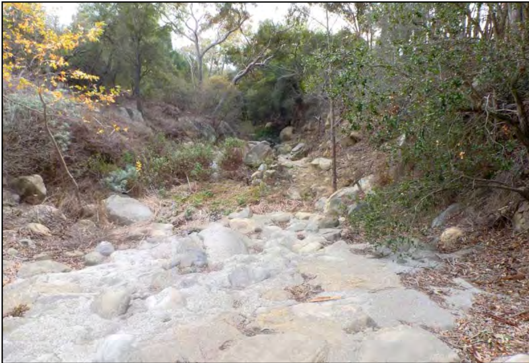
PHOTOGRAPH 5.4-1 San Ysidro Creek Debris Basin Looking Downstream
