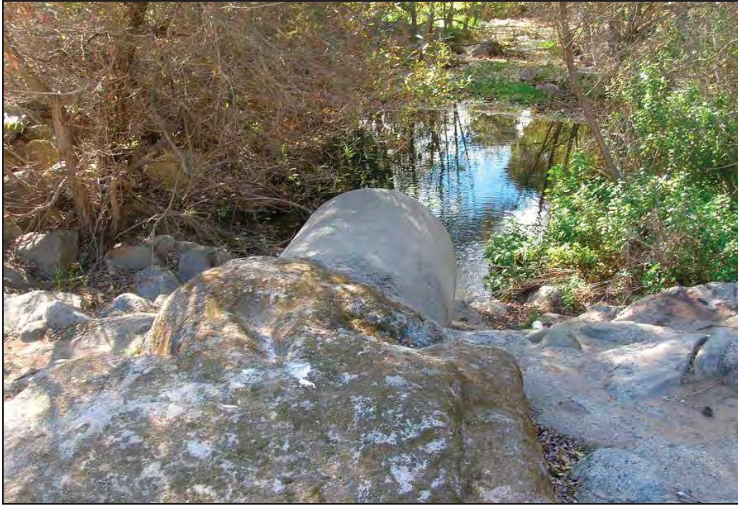
PHOTOGRAPH 4.2-3 Maria Ygnacio Creek, East Branch Debris Basin Looking Downstream
