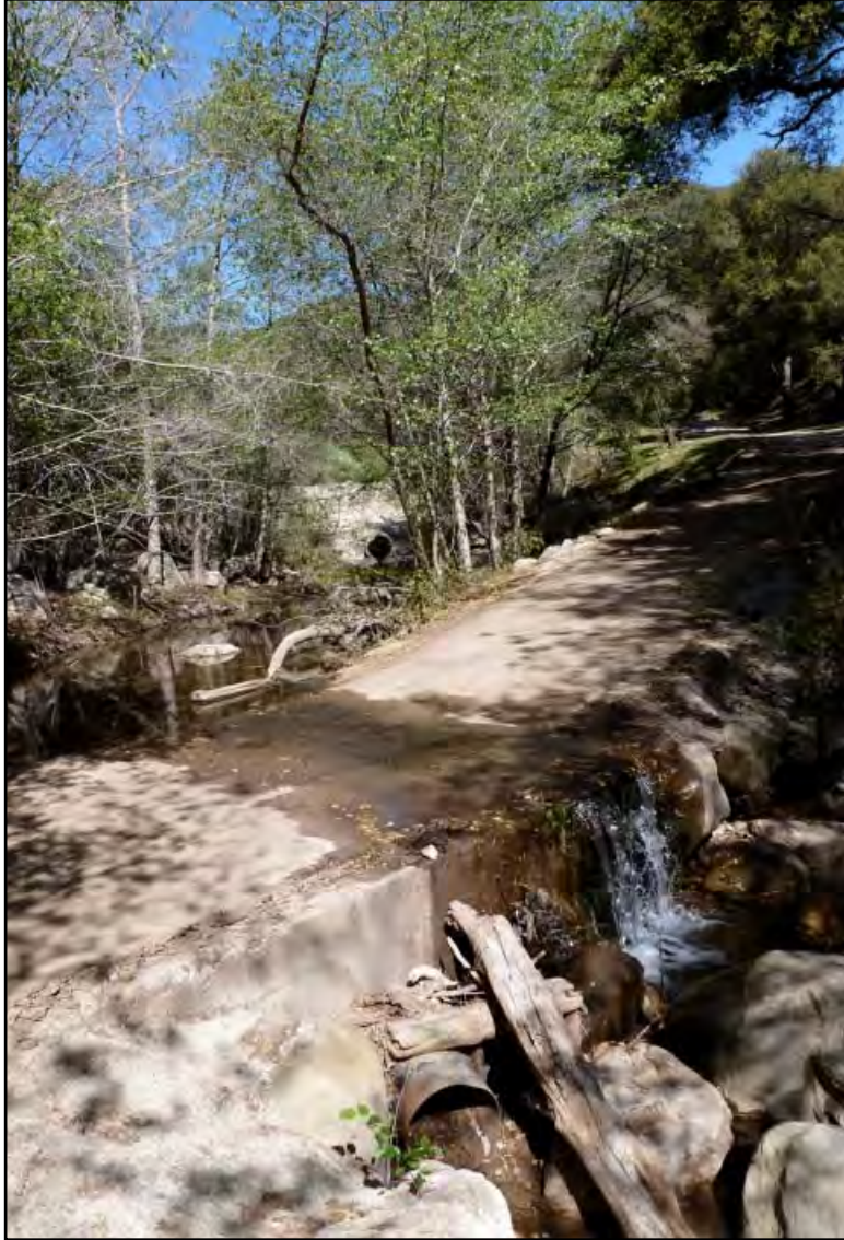
PHOTOGRAPH 4.3-4 Maria Ygnacio Creek, Main Branch Debris Basin Summer Crossing Looking Upstream
