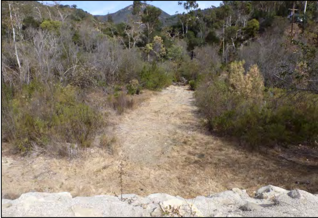
PHOTOGRAPH 4.1-1 Cold Springs Creek Debris Basin
