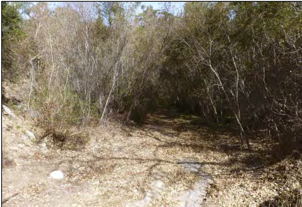
PHOTOGRAPH 5.4-4 San Ysidro Creek Debris Basin
