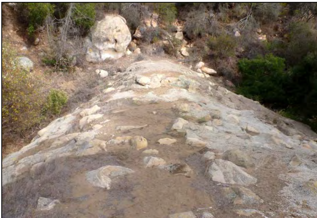
PHOTOGRAPH 4.4-2 Rattlesnake Creek Debris Basin Embankment
