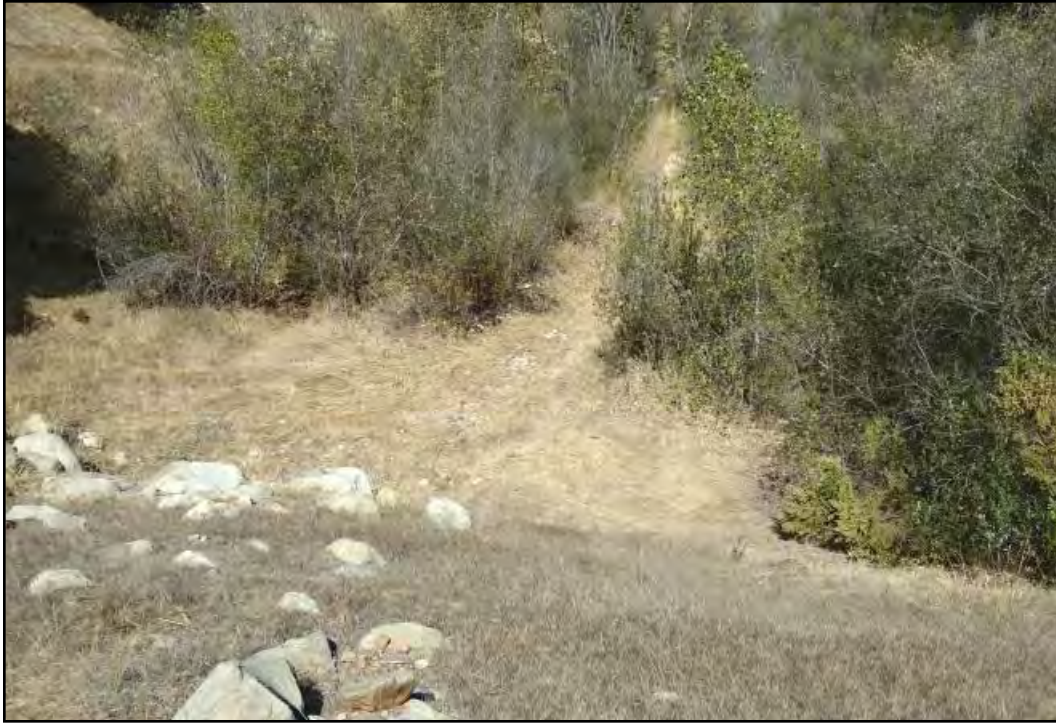
PHOTOGRAPH 5.1-1 Arroyo Paredon Creek Debris Basin
