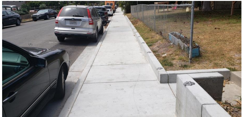
After - A portion of Trigo Road, looking west
