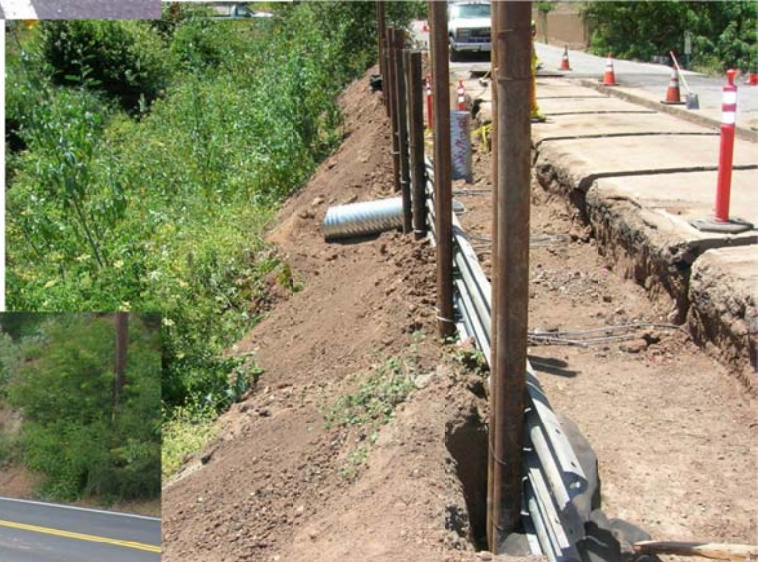
Tunnel Road at MP 0.7 (Site 1A02) while under construction
