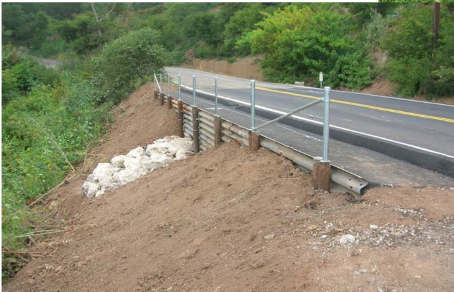
Tunnel Road at MP 0.7 (Site 1A02), Completed Retaining Wall
