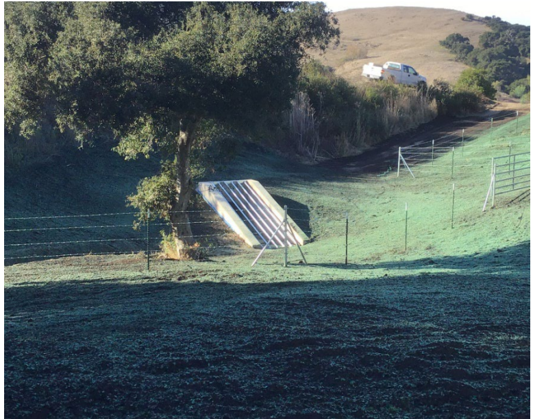
Figure 2: New Jalama Rd Culvert System
