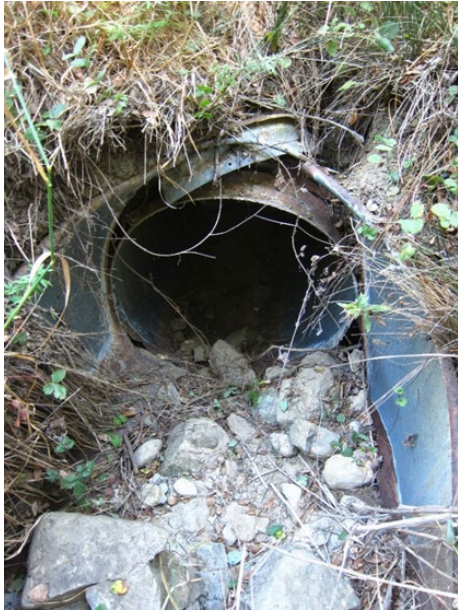
Figure 1: Original Jalama Rd. Culvert Inlet
