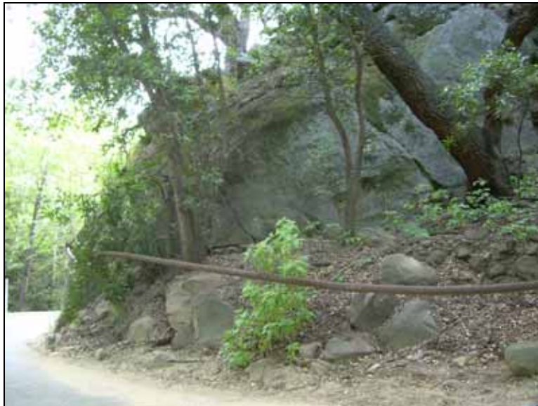
Photo: Existing Refugio Road conditions and water line
