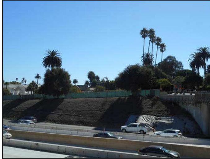
View 1: Looking south from N. Jameson Lane across US-101.
