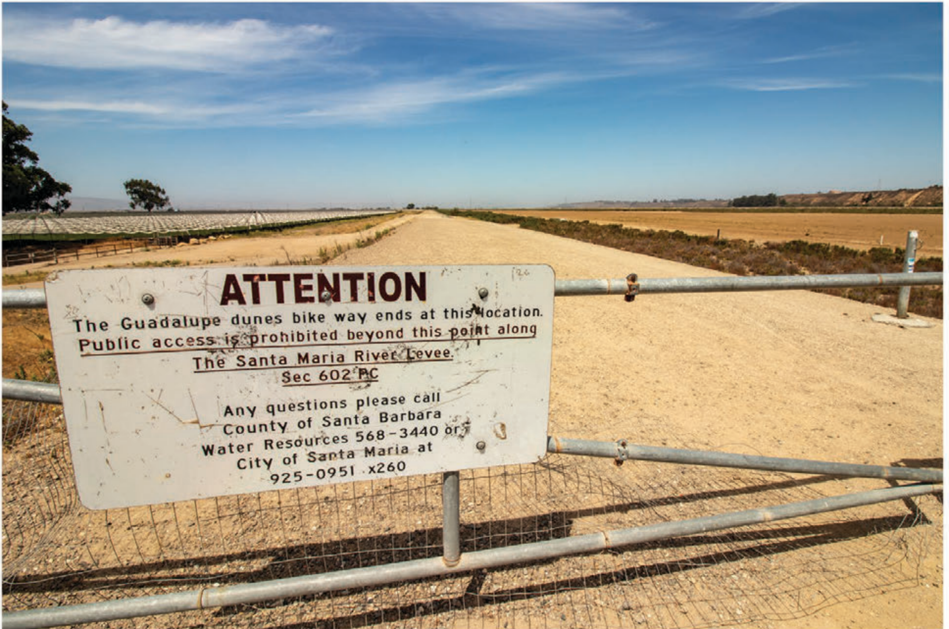
Santa Maria Levee proposed trail for improvement. Current terminus at Blosser Road. Current condition.
