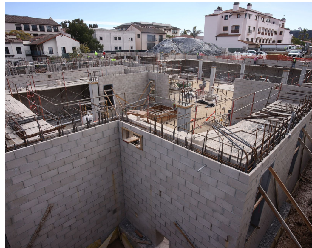
Santa Barbara Probation HQ NEW CONSTRUCTION – 4 STORY BUILDING
