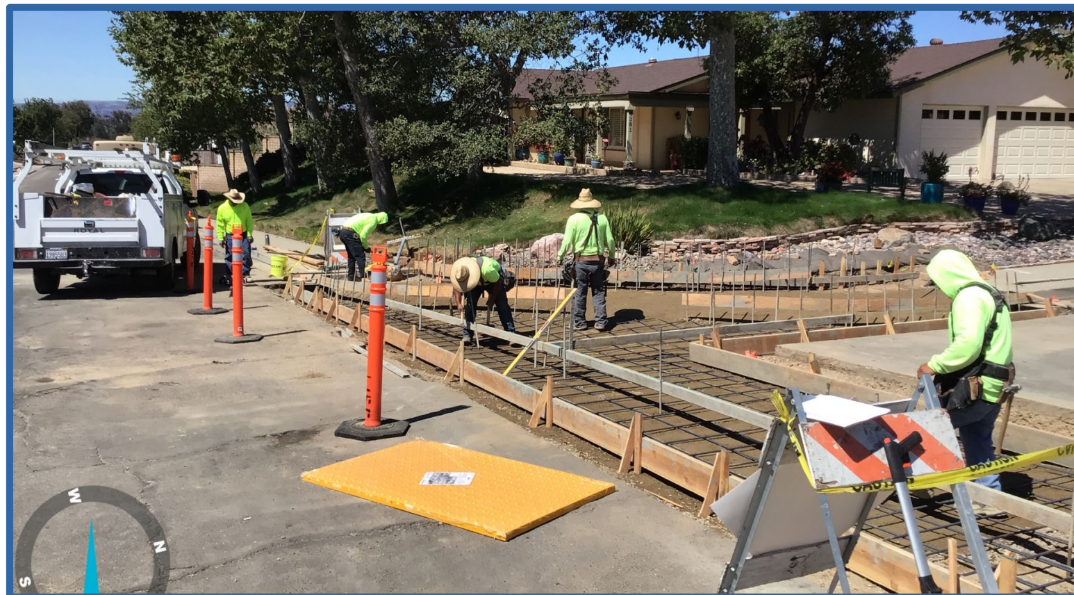
Hardscape repairs near UVP/Bradley intersection
