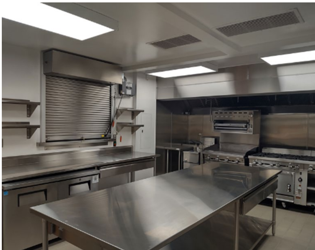
Hedges House of Hope Kitchen Renovation COMMUNITY SERVICES-NEW COMMERCIAL KITCHEN
