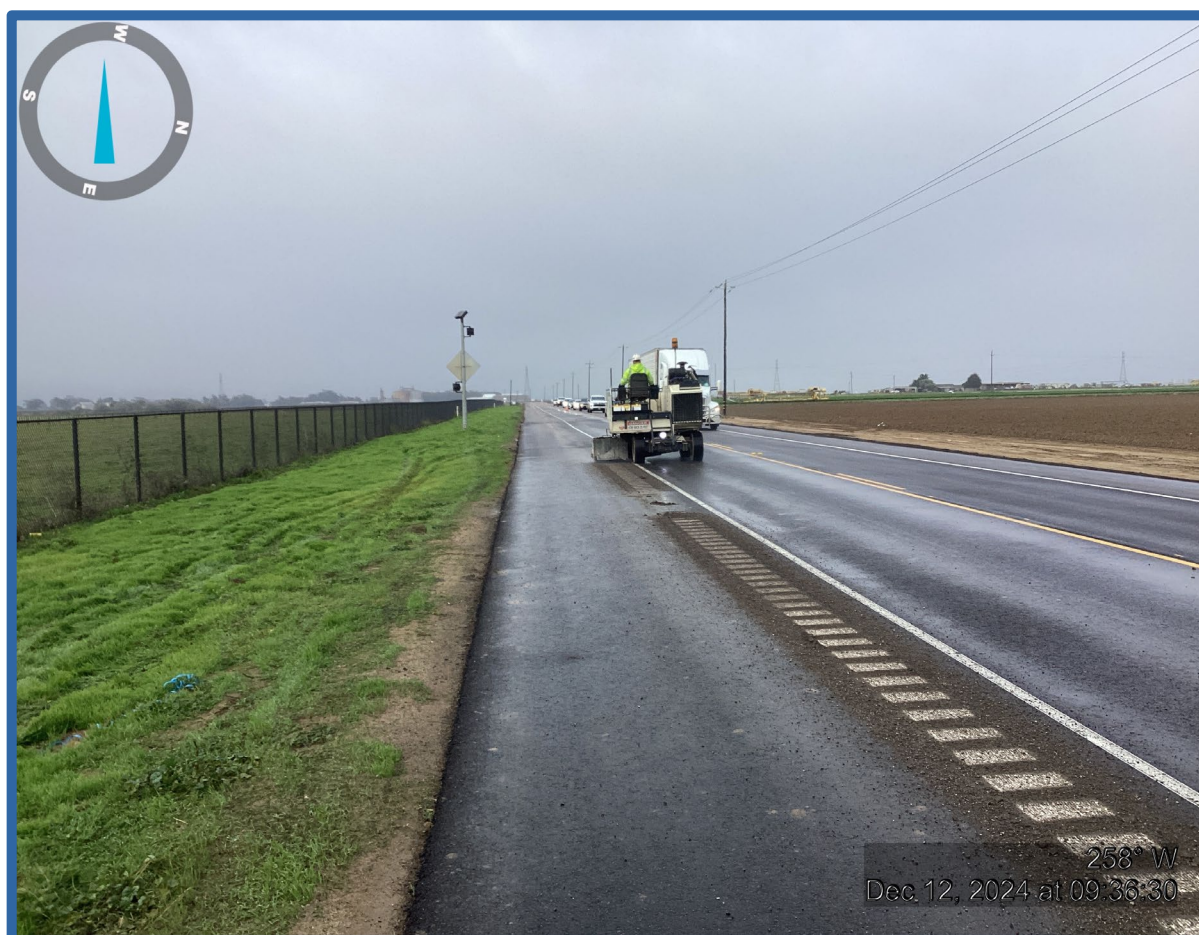
Betteravia Rd FY23/24 Rehabilitation
