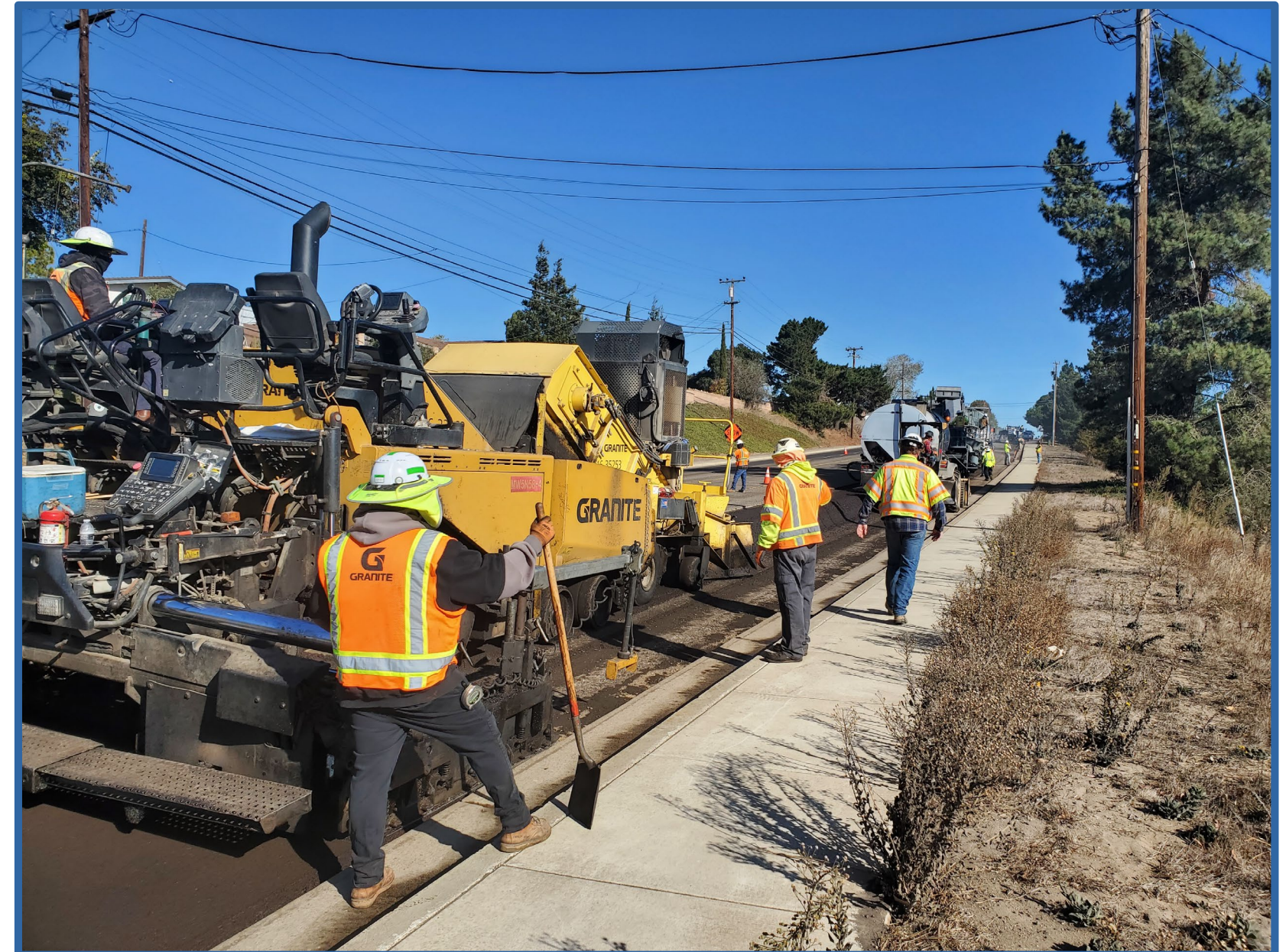
Cold In-place Recycling operations on Clark Ave
