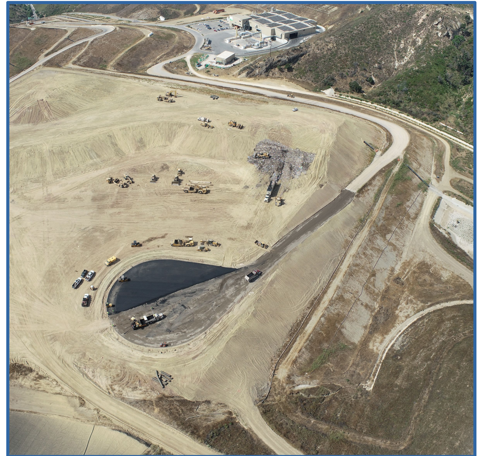
Tajiguas Landfill 2024 Access Road Extension Project
