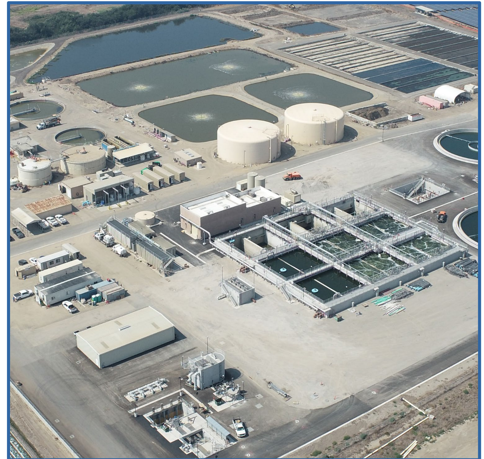
Laguna County Sanitation District Phase 1 Plant Upgrade
