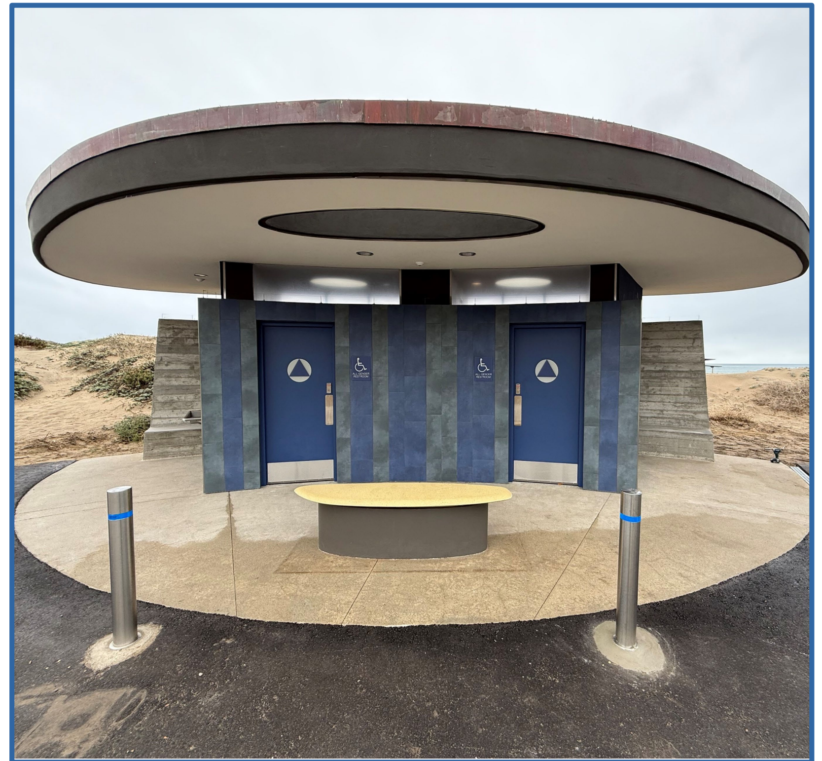
Jalama Beach Restrooms
