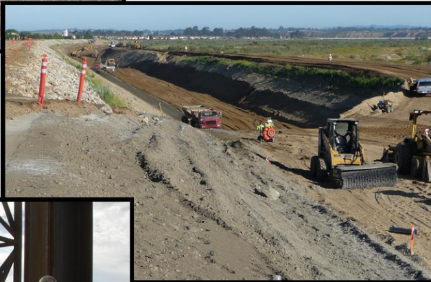
CONSTRUCTION OF SOIL CEMENT PROTECTION
