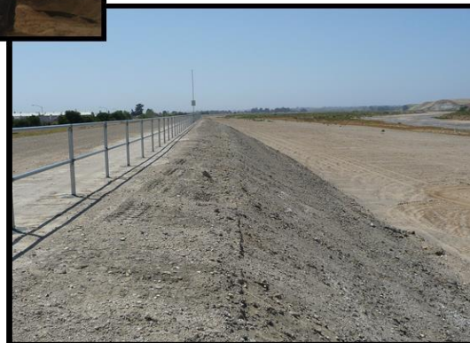
COMPLETED SOIL CEMENT PROTECTION
