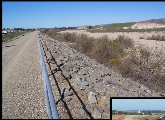
ORIGINAL LEVEE ROCK
