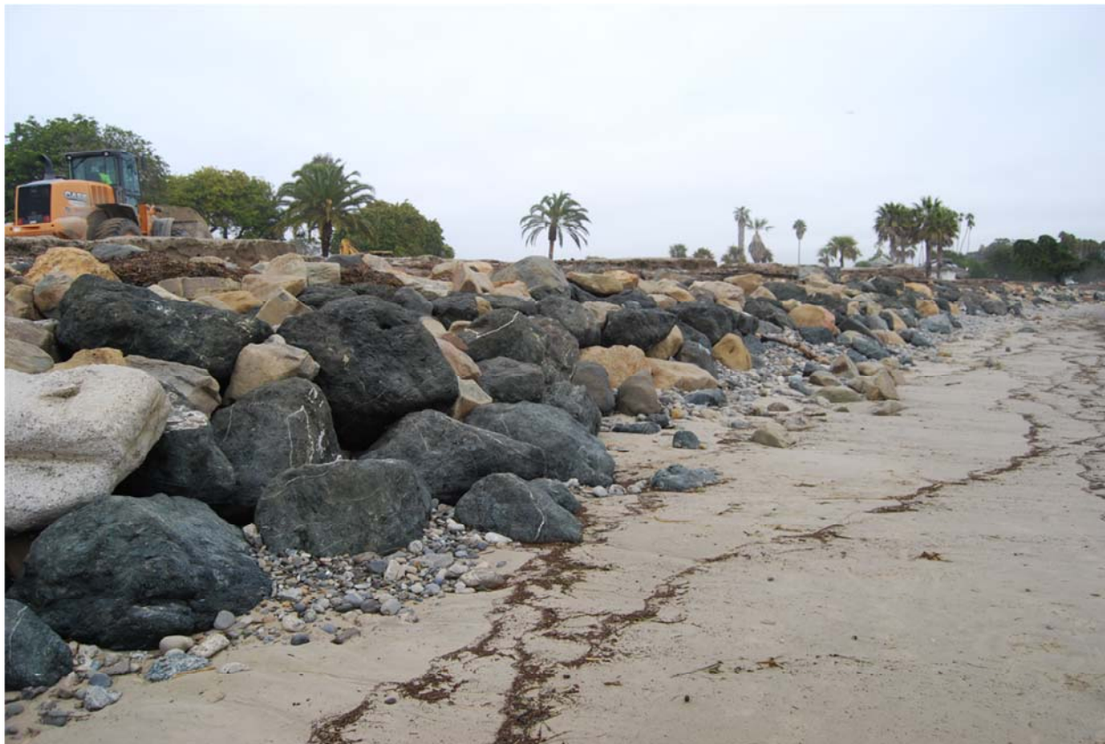
Exposed revetment at Goleta Beach in February 2017, courtesy Surfrider Foundation.
