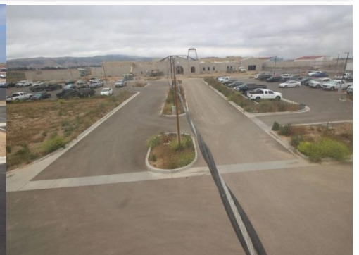
Progress Picture as of June 30, 2018
