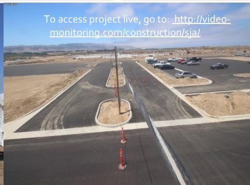
Progress Picture as of June 30, 2017
