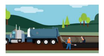
the pipe to restore its integrity. Once this is complete, welds are tested and the section is inspected to ensure repairs meet standards.
