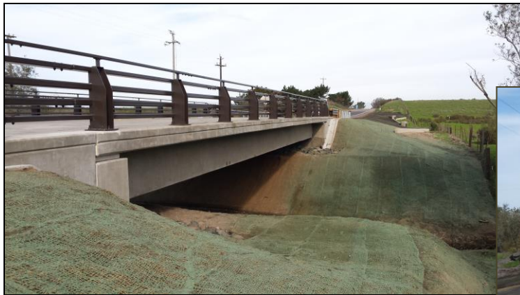
New Black Road Bridge 51C-0369
