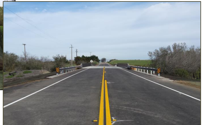
New Black Road Bridge 51C-0369 looking Northeast
