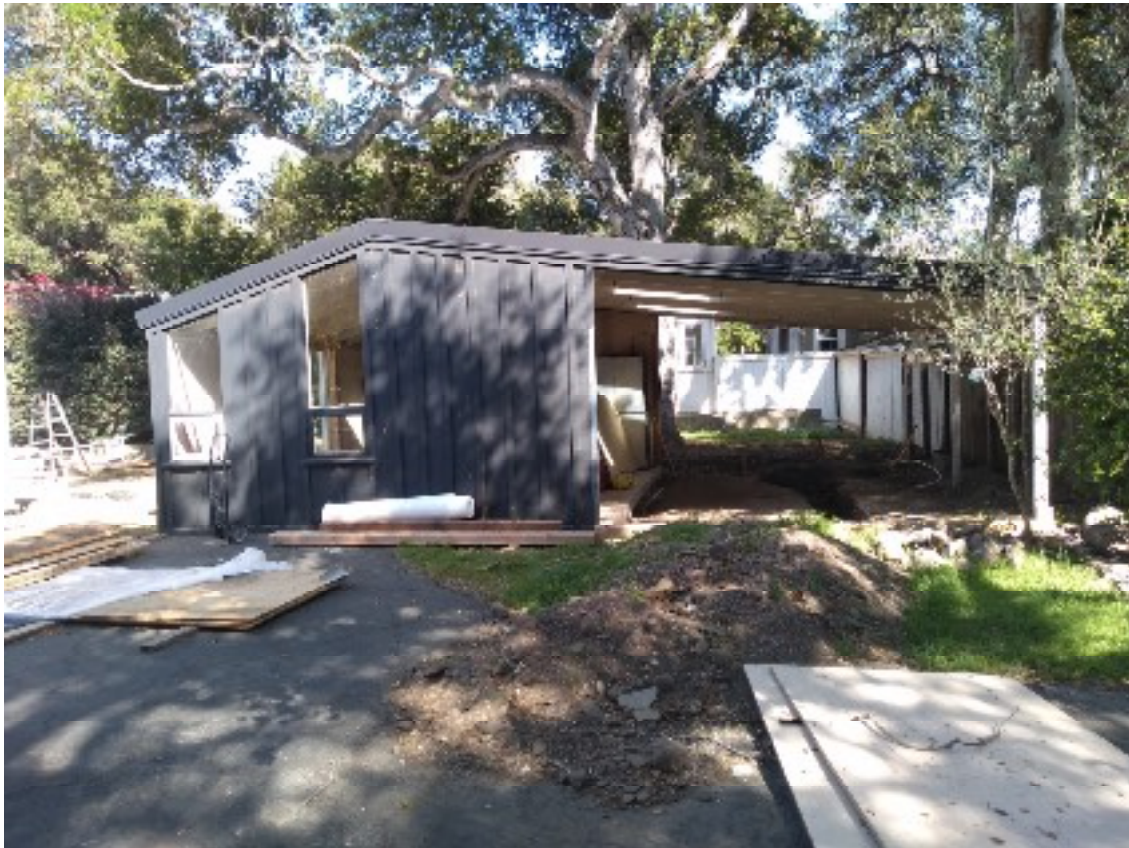
Figure 17, West elevation, looking southeast
