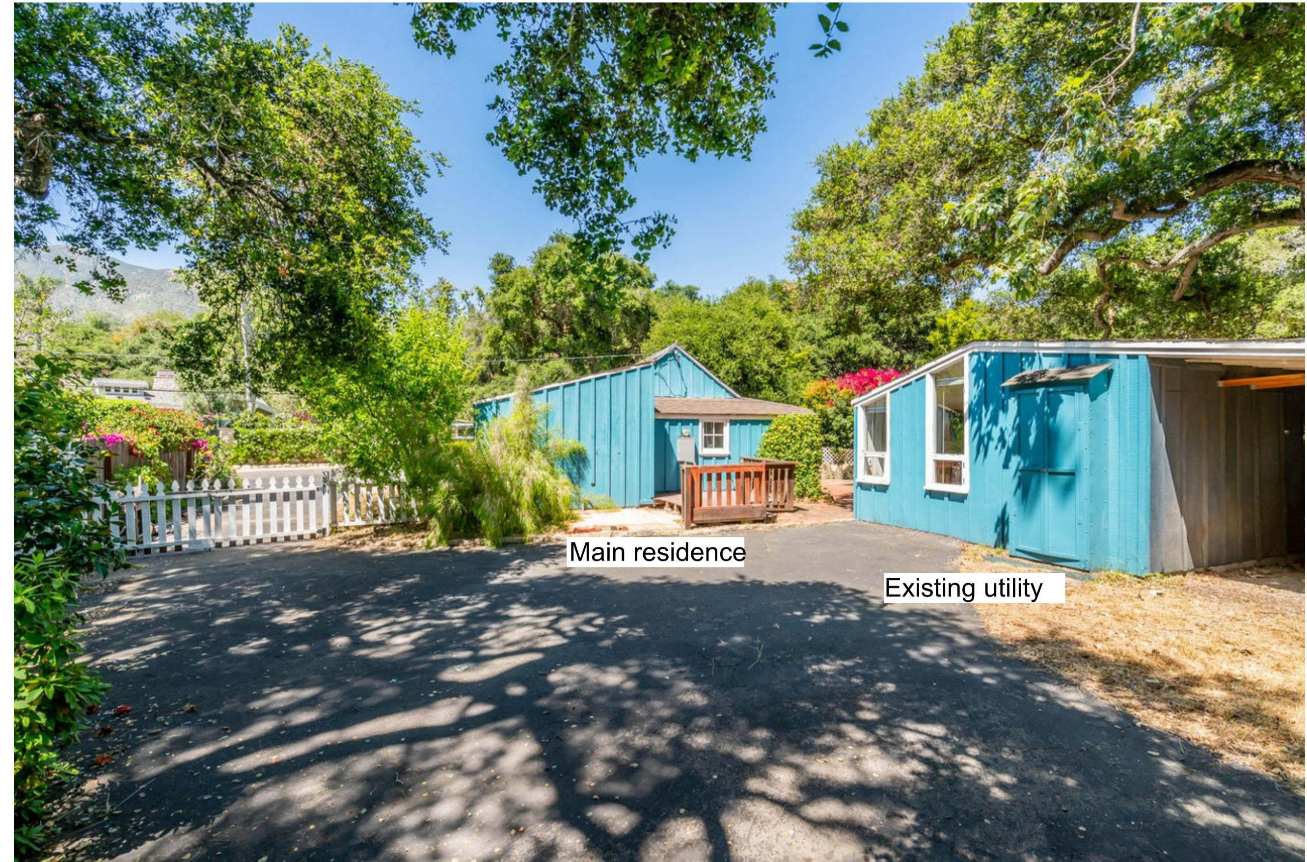
South elevation & west elevation of the utility room
