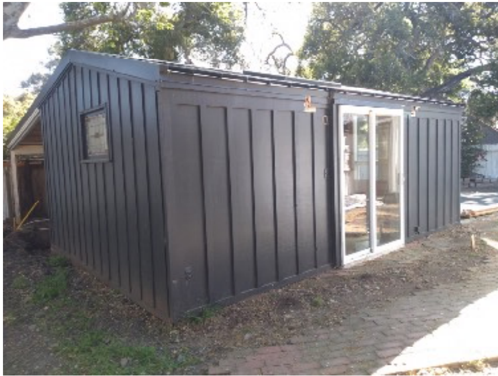
Figure 18, North and east elevations, looking southwest
