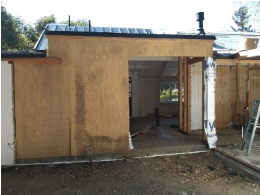
Figure 13, East elevation, looking west
