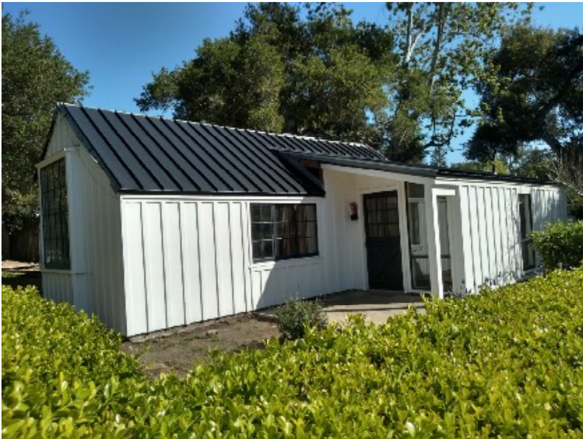
Figure 16, West elevation, looking southeast
