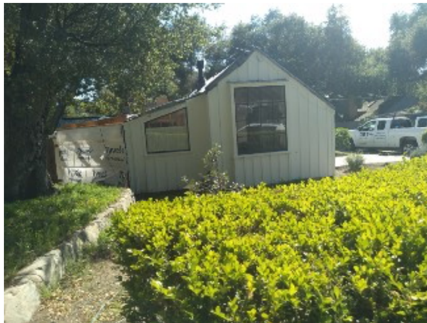
Figure 9, North elevation, looking south
