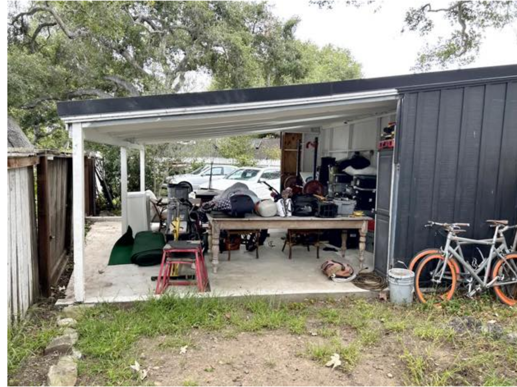
East side of Carport
