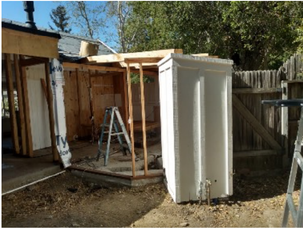
Figure 11, East end of the south elevation, looking north
