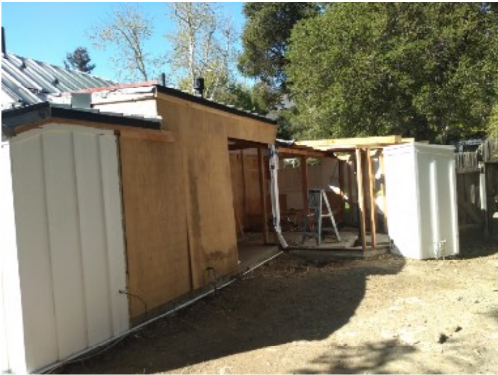
Figure 12, East end of the south elevation, looking north
