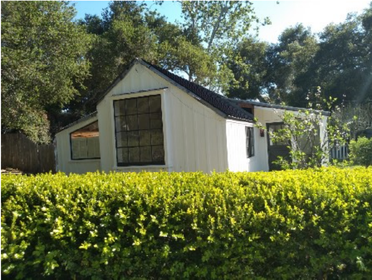
Figure 7, North and west elevations, looking south
