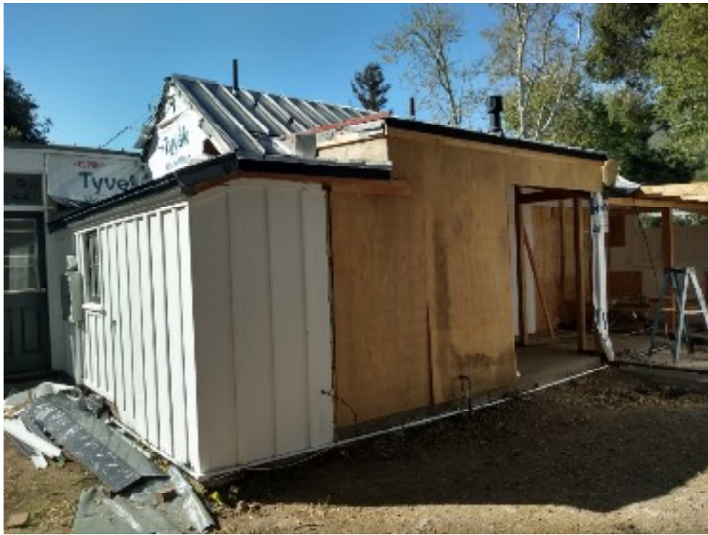
Figure 14, South end of the east elevation, looking northwest
