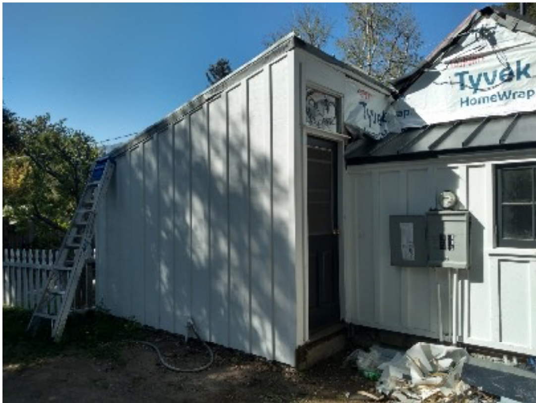
Figure 15, Partial south elevation depicting door on east elevation, looking north
