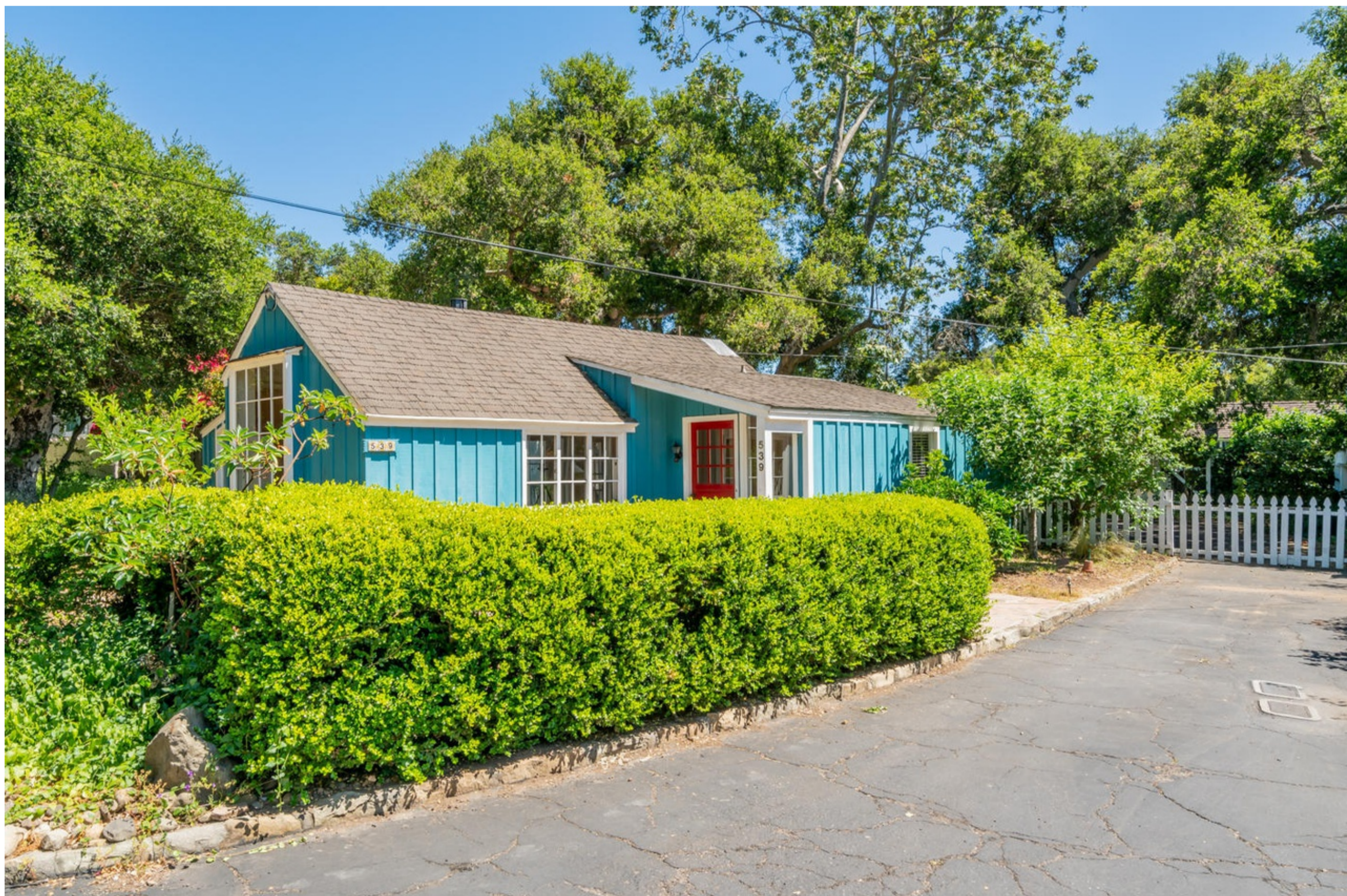
West elevation / side of the main residence
