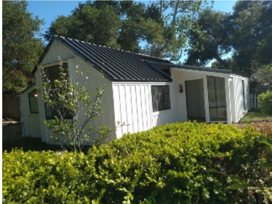
Figure 8, North and west elevations, looking south
