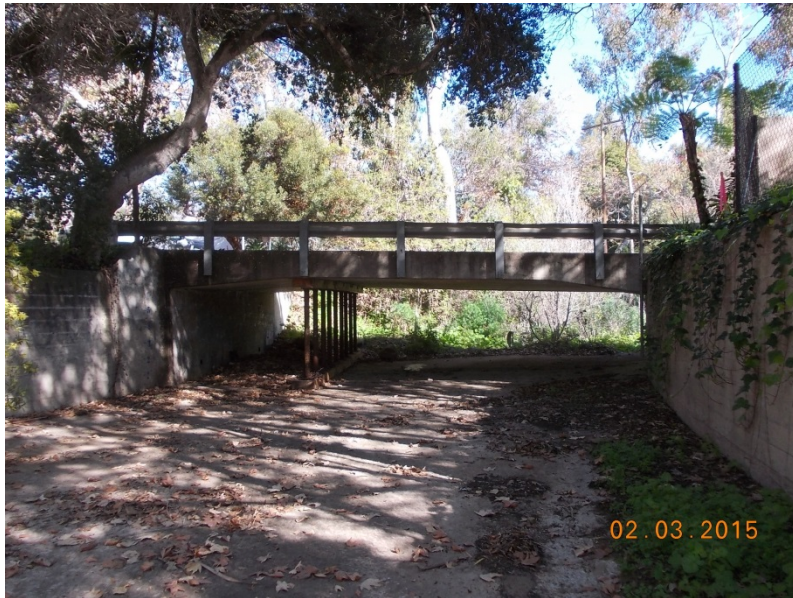
a. Existing Fernald Point Lane bridge, note temporary shoring
