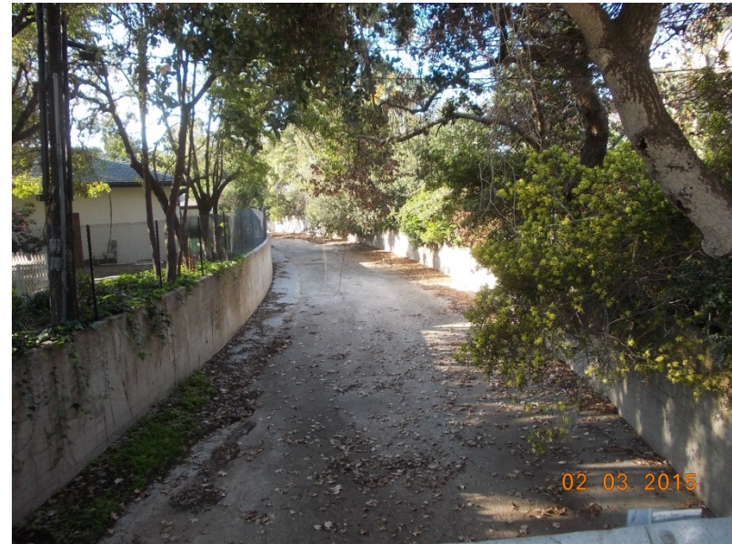
b. Rectangular concrete channel downstream of the bridge
