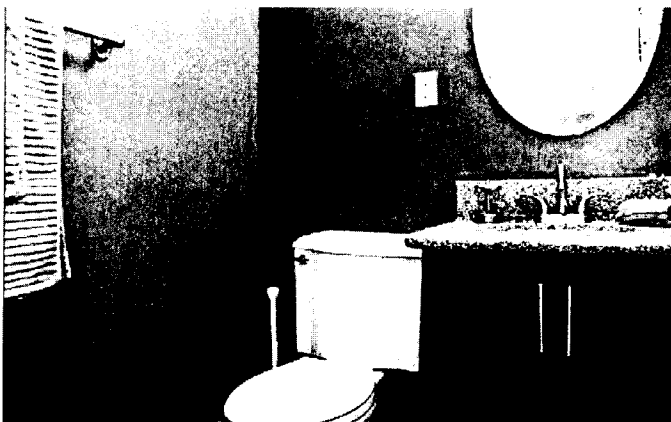
Figure 6: An AirBnB bathroom in a building with more than five units. There are no grab bars in this bathroom.
