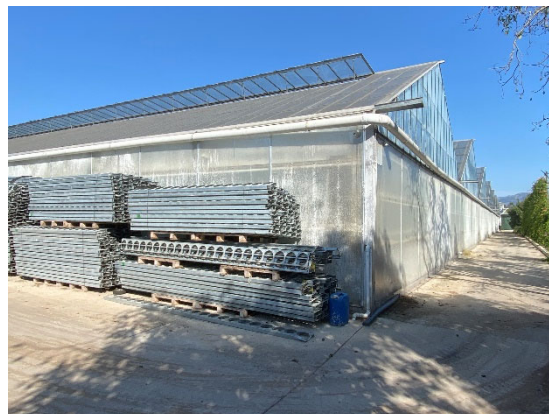
Figure 3- Existing Greenhouse Exterior & Roof Venting
