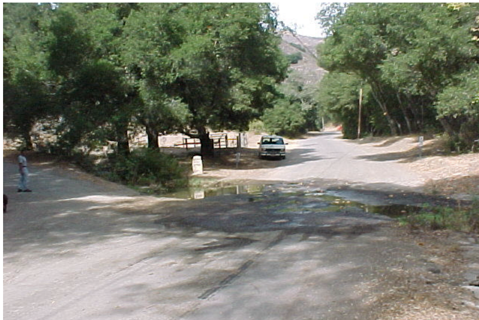
Photo: Existing Tepusquet Crossing conditions (10/11/2001)
