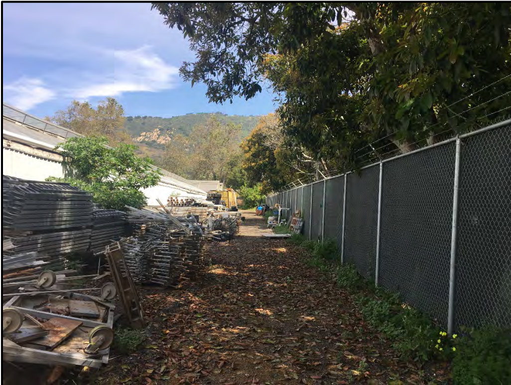
Photo 4: East side of Project Site where underground stormwater detention basin will be located, outside of the ESH buffer (Aspect: North). Photo taken 5/7/2020.
