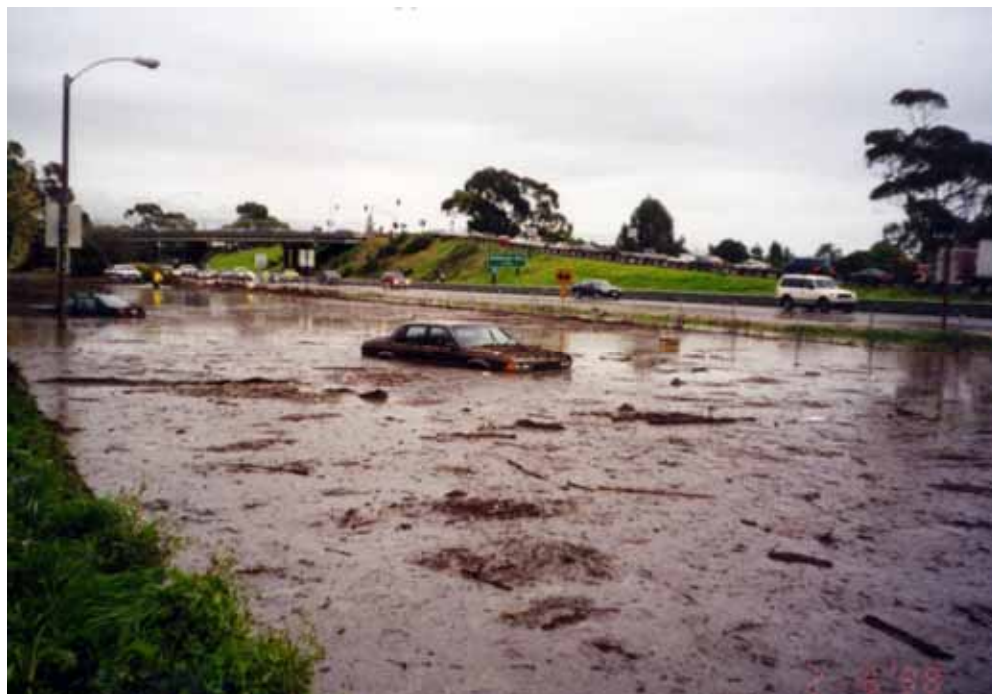
February 1998 Storm - Calle Real @ Fairview
