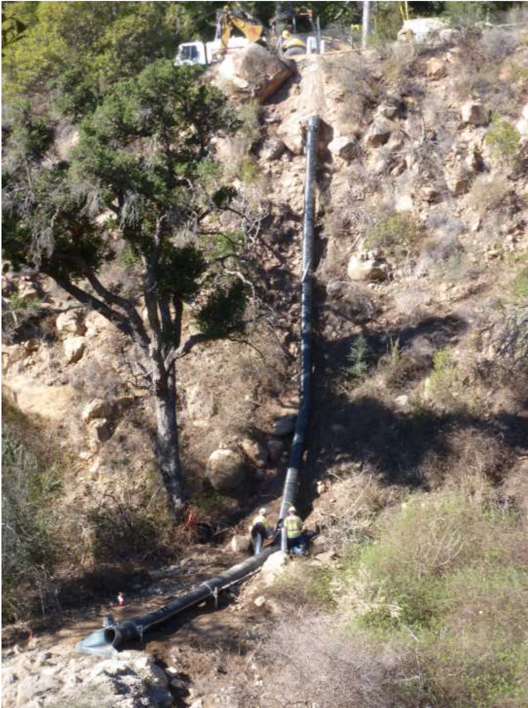
Mission Creek Debris Basin Storm Drain Project – Tunnel Road Downdrain
