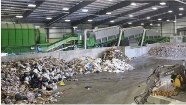
WM San Antonio Mixed MSW Dirty MRF Recycling & PEF- Pellet constructed in 2011
