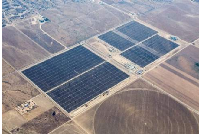
Figure 2.2: Aerial View of 40 MW Cuyama Solar Array
