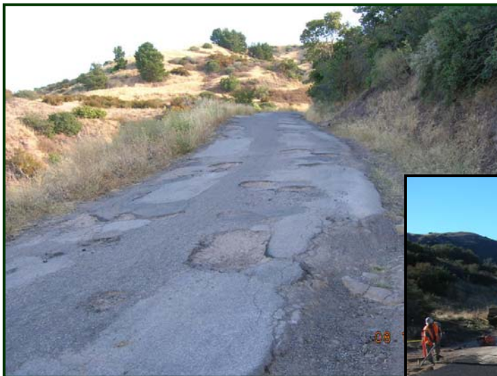
East Camino Cielo Before Construction
