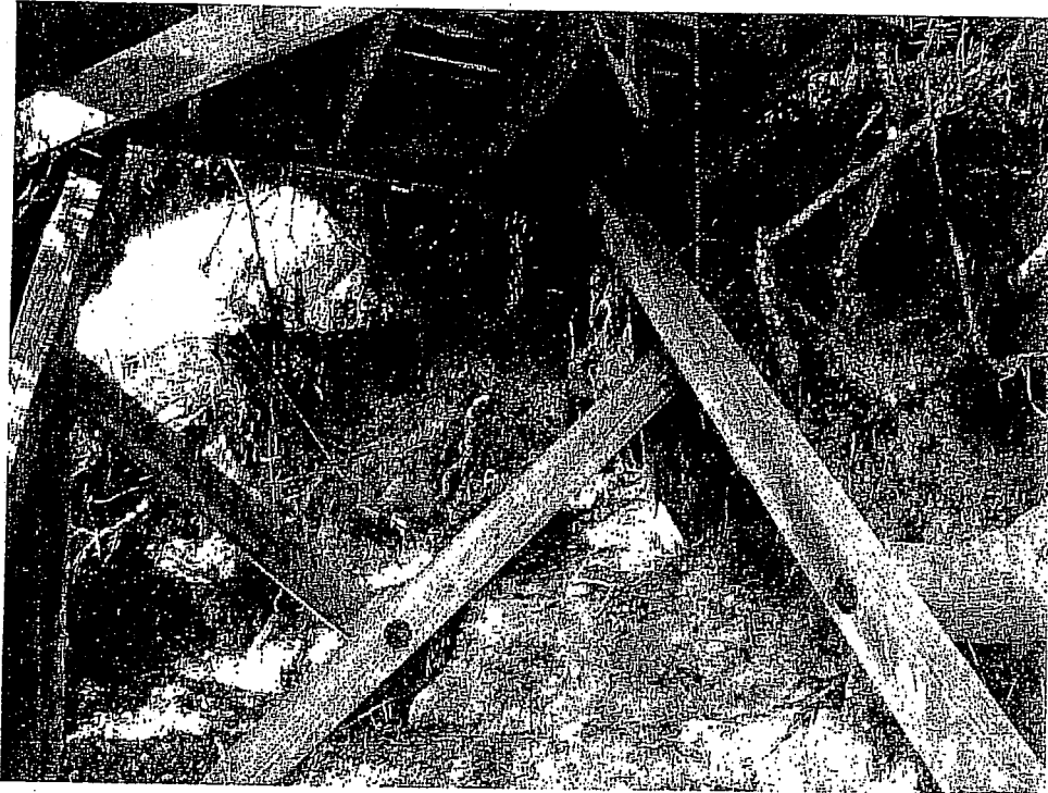
Shallow Slope Sloughing Causing Pier Deflection Under Middle Landing of Staircase
