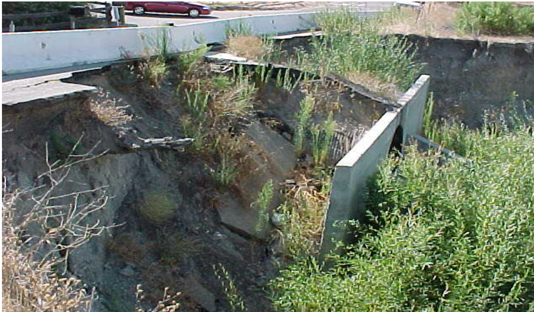
Photo: Existing Ballard Canyon Road Conditions (08/16/2001)
