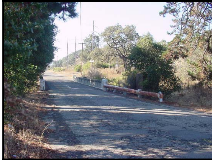
Photo: Existing Bridge 51C-0225 Jonata Park Road (Looking South)
