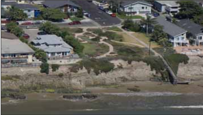
Photo 2: Southerly terminus of Camino Pescadero
