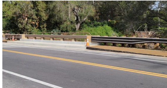
Hot Springs Road Bridge Rail Repair, Bridge 51C-041
