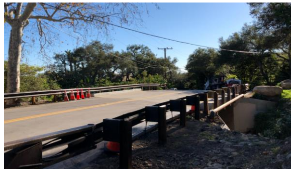
Lilac Drive Bridge No. 51C-200
