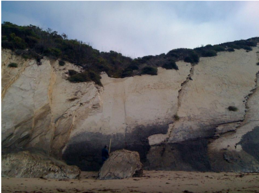
Photo C: Unnumbered Local Drainage between #4 and #5
