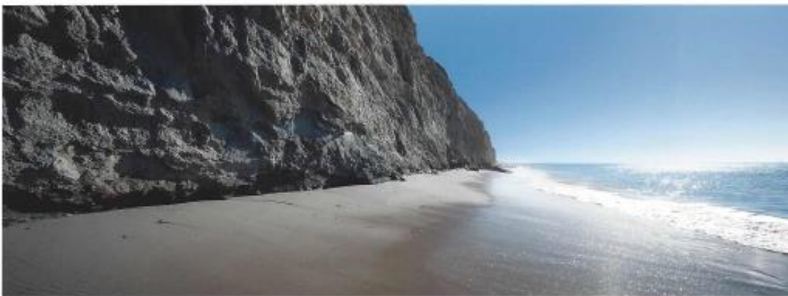
Summerland Beach Looking East Note dangerous nature of bluffs.
