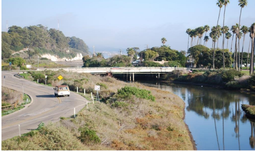
Existing Bridge 51C-0158
