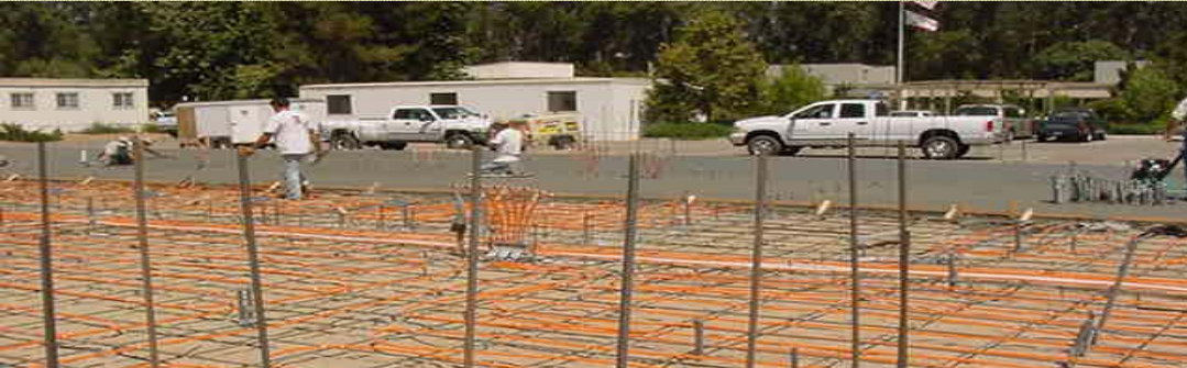
Radiant Floor Heating (can be retrofitted to use excess energy from Juvenile Hall HVAC system)
