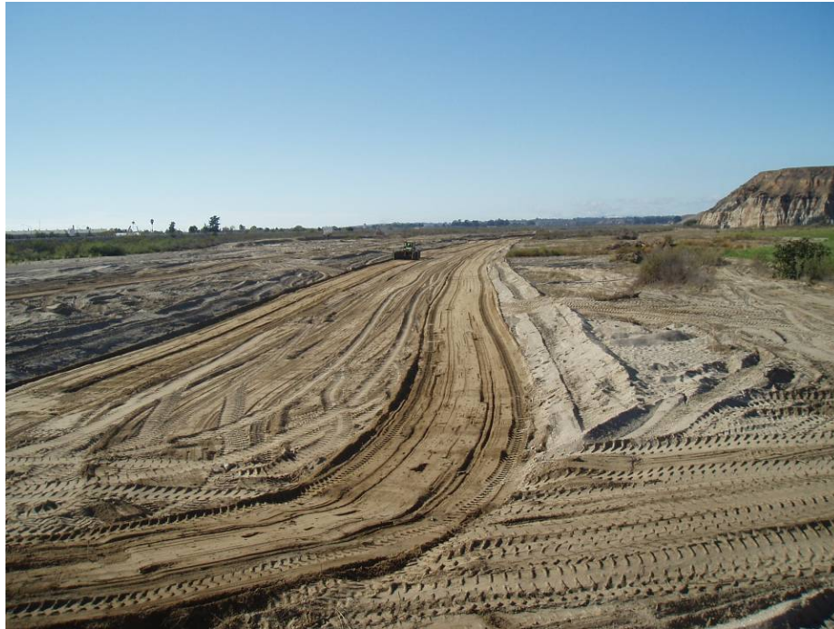
Figure 4 – Pilot Channel Construction at Suey Road, Santa Maria River
