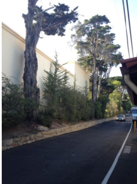
Potential location for Verizon Wireless treepole at Verizon switch
