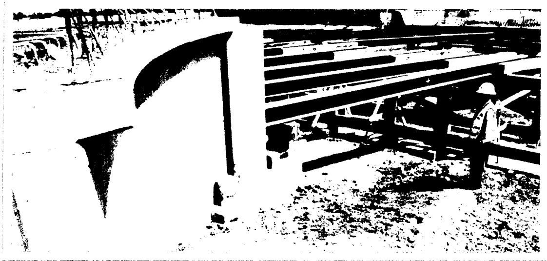
Md. Wahiduzzaman inspects the bridge foundation and falsework for the Cohansey Ave. Bridge. Note flared wing walls.
