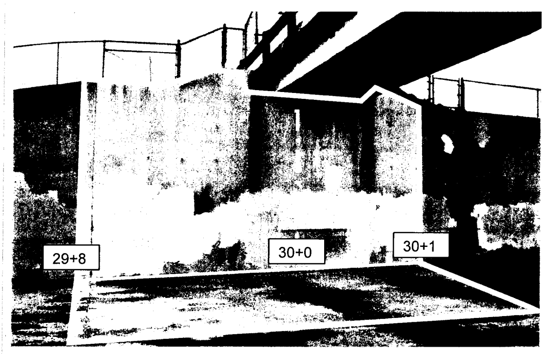
View of the West Abutment of the existing spillway bridge. The existing bridge abutments, (highlighted) are structurally different than the adjacent channel walls.
