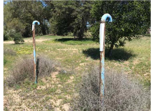
**Photograph 6.** View of two vent pipes located in the southwestern corner of the subject property.
