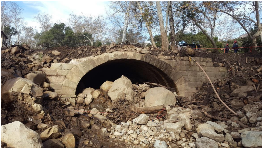
Ashley Road Bridge – Looking upstream
