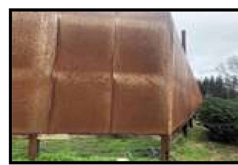
C POST & STEEL FENCING
