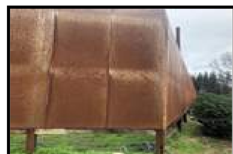
C. POST & STEEL FENCING
