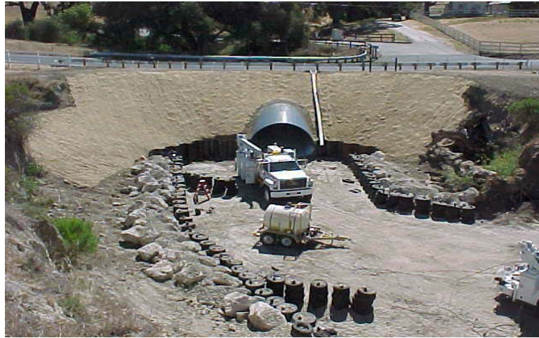
Photo: Existing Ballard Canyon Road Conditions (06/18/2002)
